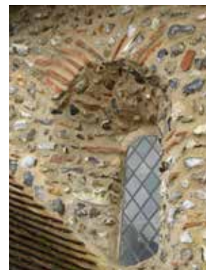
Roman tiles forming a double-splayed nave window at West Barsham
