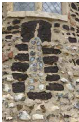
left: window of conglomerate blocks in the tower at Beeston St Lawrence
