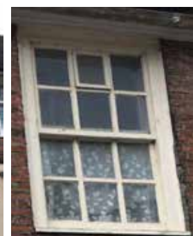
Burnham House, 13, Nelson Street, Lynn. Opening lights set within the sash windows
