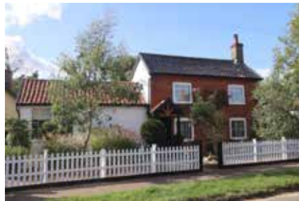
Bay Trees - similar to, but smaller than, The Laurels with a single chimney and a clay-lump addition to the south.
