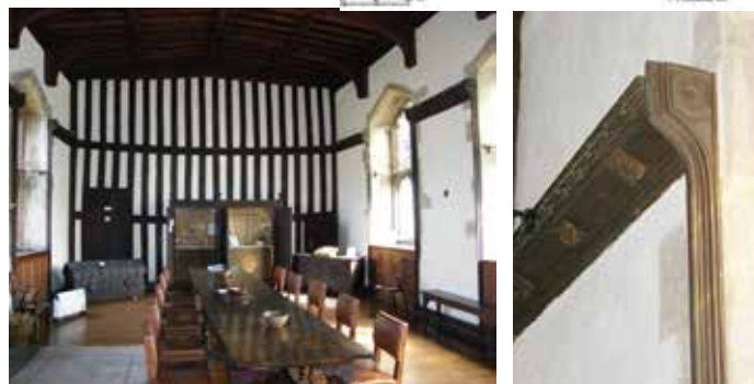
The first-floor Audit Room and the cornice for the wall hangings, seen on the right of the main image
