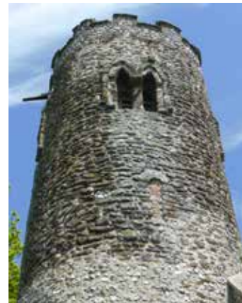
The belfry window with strip-work above it at Bessingham - below it is a bricked-up loop with a monolithic head carved from a block of conglomerate
