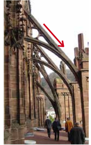
At Freiburg Cathedral, the thin flying buttresses follow the direction of the combined force
