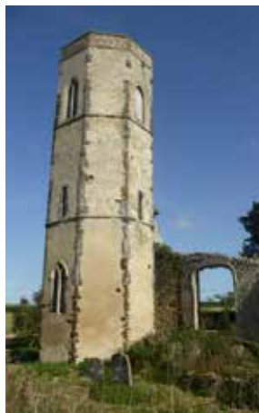
Edgefield tower with conglomerate quoining
