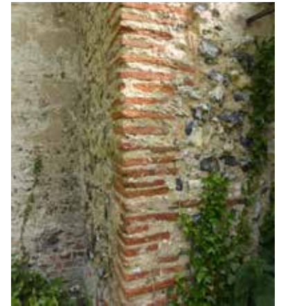
right: The western quoins of Oxnead St Michael are composed entirely of Roman tiles, probably from Brampton sited just across the River Bure
