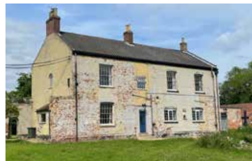
The rear elevation showing two casement windows as well as four of the same sash windows as the front
