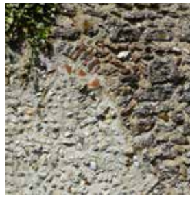
Swanton Novers - blocked south doorway with an arch of reused Roman tiles defining its top
