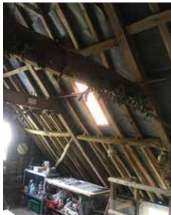
North plane of the roof
