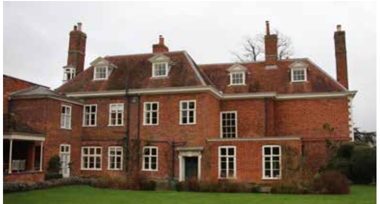
The rear of Cavick House with signs on the brickwork of a reversed staircase on the right of 1720s house. Late C18 kitchen extension on right. 1953 loggia at left.
