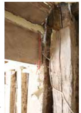
Side-by-side posts between the parlour and stack
