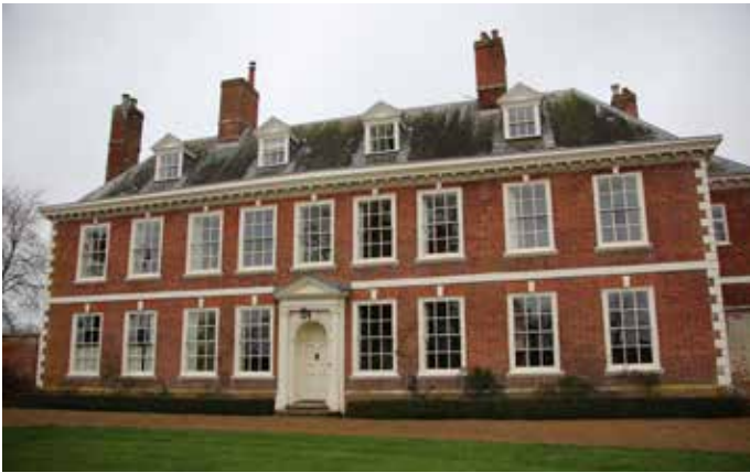
Frontage of the house- central five bays with two later bays at each side. Renewed attic windows. Central door with engaged doric columns and pedimented hood.
