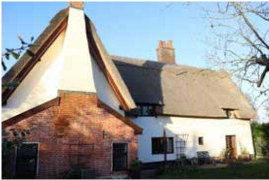
The external chimney on the south gable of the crosswing which covers a window on the second floor
