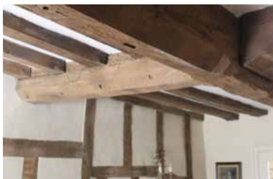
The large crossed ceiling beams in the centre of the original building
