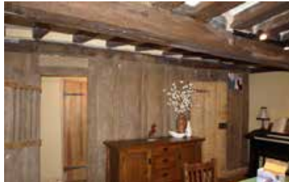
Elm Tree Farm - plank & muntin cross-passage screen / subsidence on moat side
