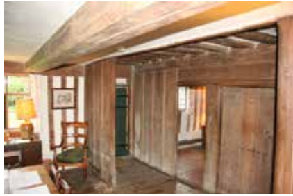
Manor Farm - plank & muntin cross-passage screen / original shutters of 1615
