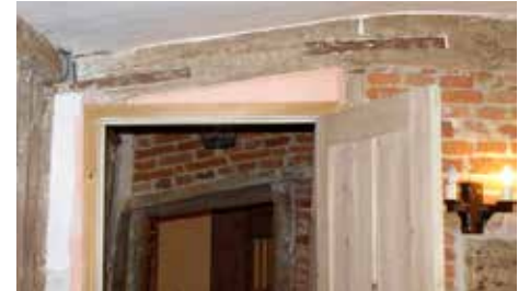
Elm Tree Farm - plank & muntin cross-passage screen / subsidence on moat side
