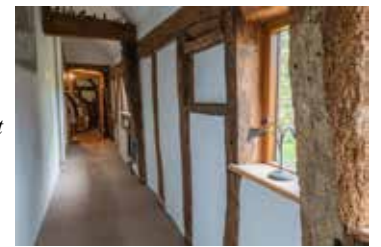
Large section timbers through
