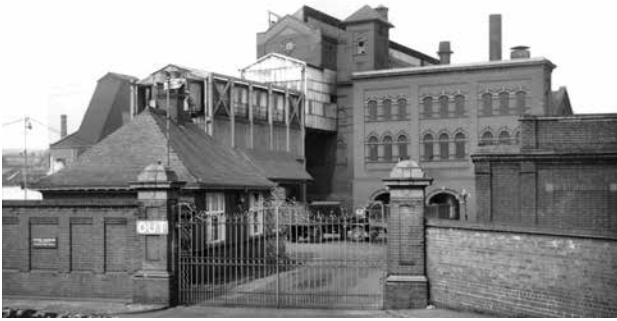
The gasworks on St Martins Palace Plain © George Plunket Collection
