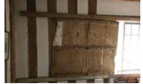
Manor Farm - plank & muntin cross-passage screen / original shutters of 1615
