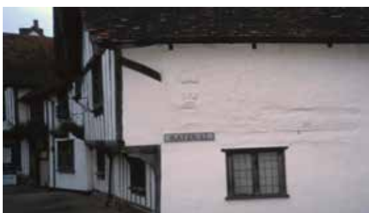
Remnants of pargetting in Lavenham, Suffolk, probably not well-enough off in the 19th century to have a new brick facade
