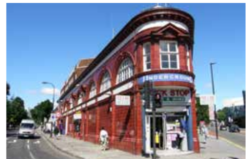
Chalk Farm - 1907 Leslie Green, UERC - The Charing Cross to Hampstead Railway, built on a difficult site
