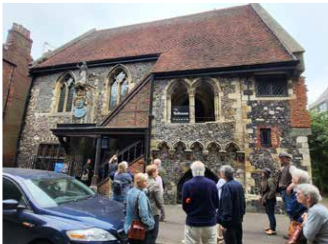
The Tolhouse north facade
