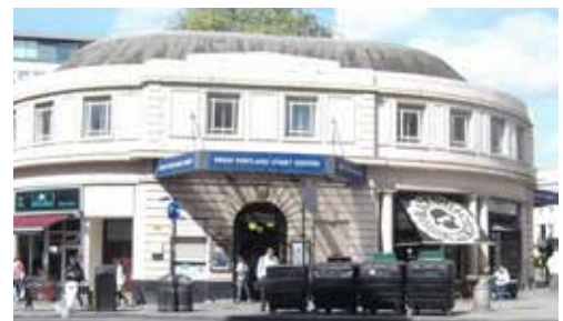
Great Portland Street - 1930 Charles Clark. Metropolitan Railway station rebuilt in 1930 - modernism beginning to creep in for Met Rlwy.
