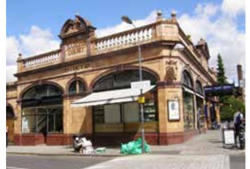
Barons Court - 1905 Harry Ford, District Railway. Built in preparation for the opening of the Great Northern, Piccadilly and Brompton Railway
