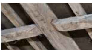
left: half dovetail and carpenter's marks
