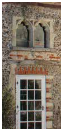
The remains of the two nine-foot tall hall windows in the front and rear walls. The top of the rear windows still display the original glazing groove
