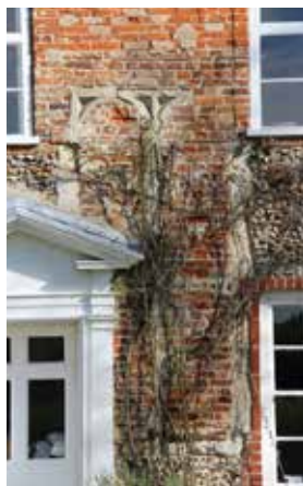
The remains of the two nine-foot tall hall windows in the front and rear walls. The top of the rear windows still display the original glazing groove
