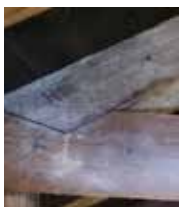
left: half dovetail and carpenter's marks
