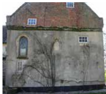
right: The glazed doorway in the northern gable end indicating that the building was once longer
