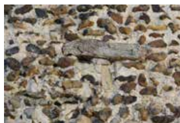
one of the two timber putlog-hole lintels for the medieval scaffolding when the house was first built
