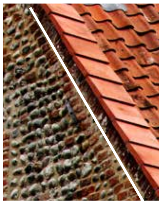
Bessingham Manor Farm - Left: two gable raises Right: final gable raise above the half bricks on the right side, additionally protected by modern capping tiles
