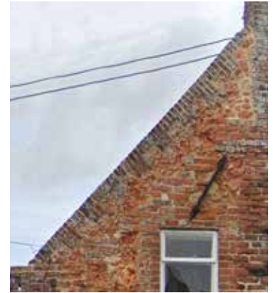
Brick-on-edge gable end at Church Road, Hunstanton - not using tumbling-in, but imitation rustication.
