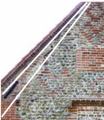
Bessingham Manor Farm - Left: two gable raises Right: final gable raise above the half bricks on the right side, additionally protected by modern capping tiles
