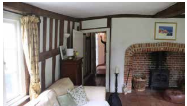
The parlour brick fireplace with one of the blocked original mullion windows on the left
