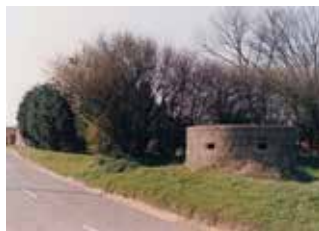
A hexagonal pillbox, cast-in-situ. A pair of these guard the A47 near Yarmouth
