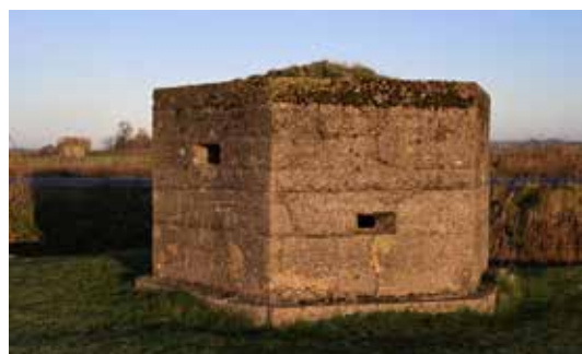
A hexagonal pillbox, cast-in-situ. A pair of these guard the A47 near Yarmouth
