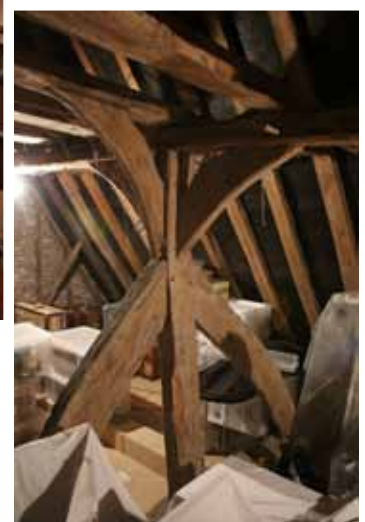
The wall-post and brace supporting the tie beam on which the crown post sits
