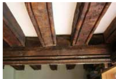
and roll-moulded principal and common joists in the hall
