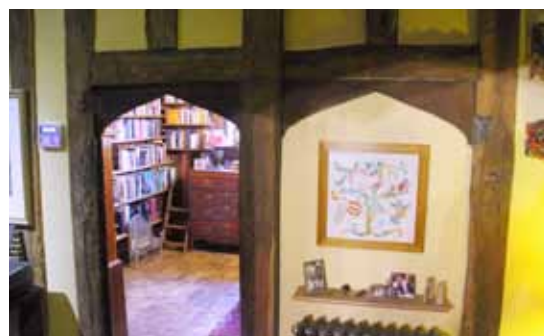
The two spandrelled service doors leading off the cross passage
