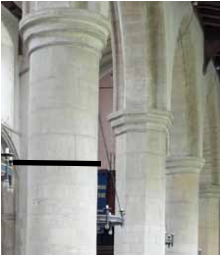
The Norman piers, extended upwards in the 14th C above the black line shown above photo: Richard Ball
