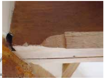
H - Fig 6 from Abbot Lowell Cummings' book - showing the principal joist as resting on an inserted timber, rather than moticed in.
