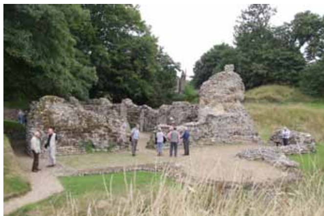
The east end of the chapel/palace ruins taken from Despenser's earthwork bank photo: Maggy Chatterley
