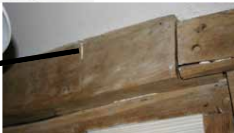
J - right Face halved and bladed scarf joint with error, at Burrage House, New Buckenham
