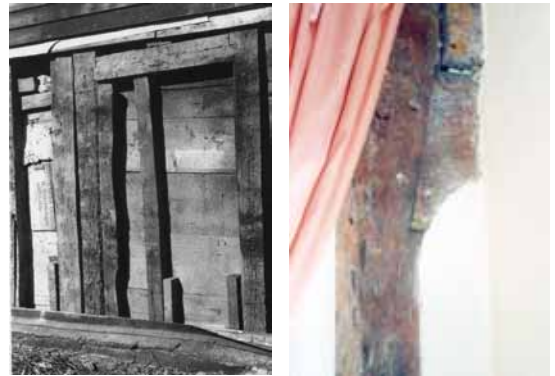
A - Doorhead - Fairbanks House - Blair House. New Buckenham
