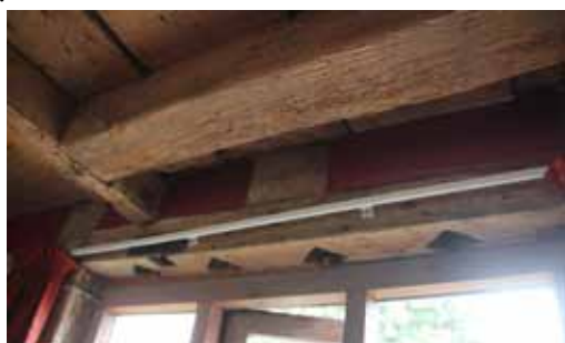
empty diamond-mullion sockets and flat-laid joists
