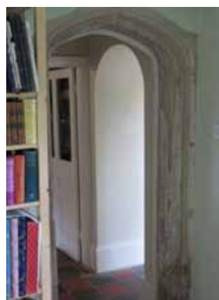
four-centre-arched doorway into original cross-passage?
