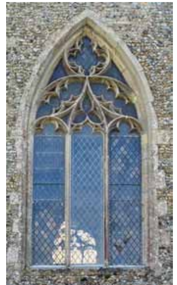
St Mary's, Elsing and its curvilinear window tracery
