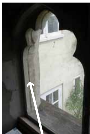
Glazing groove in the two-light windows
