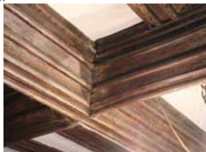
Roll-moulded principal joists, with moulded common joists - 1520?
