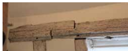
edge-halved, bridled scarf joint with shutter slide
