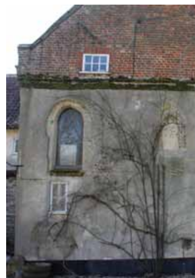
First-floor opening in the north gable
