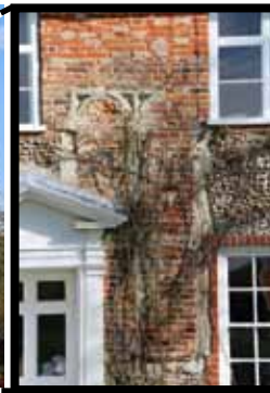
left: west elevation - INSET showing the remains of the hall window
