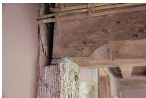
tenonless principal joist resting on a cut-out
