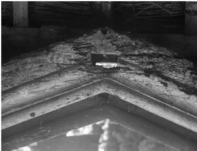
Central camber beam. (see Figs. 5 and 6)
