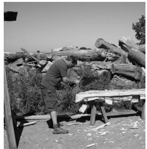
Left: a Nuremberg Housebook of 1533 shows timber having been notched and the hewing commencing, note framing in the background. Right: the same happening last summer
