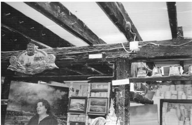
Smoke House: believe it or not, real ships' timbers gathered from Yarmouth Beach over the years.
