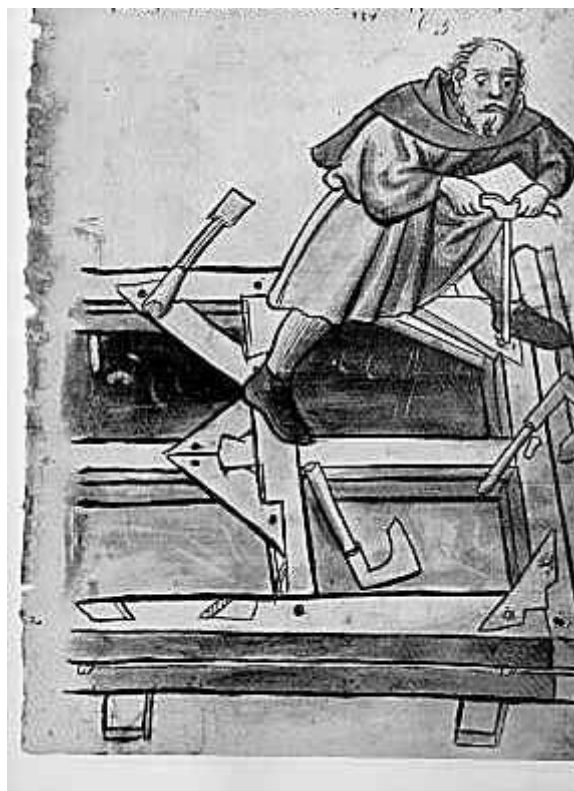
Fig. 1 German illustration from 1446, a wall frame is completed and the brace peg holes are drilled. Note that it is laid over another previously completed frame that sits on packers.
