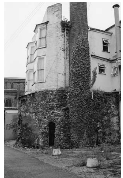
Two aspects of the walls being recycled. There is certainly a definite record of a change in the building history in the one tower on the right.
