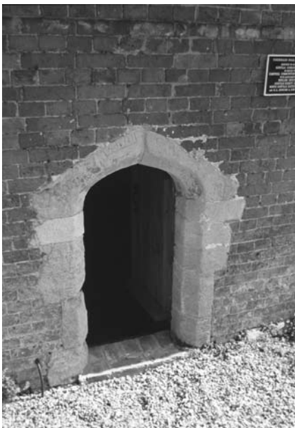
The doorway at Thornage Hall is only 4 ft 6 ins high, as in most early dovecotes, so that the pigeon-keeper could block it with his stooping body as he entered.
