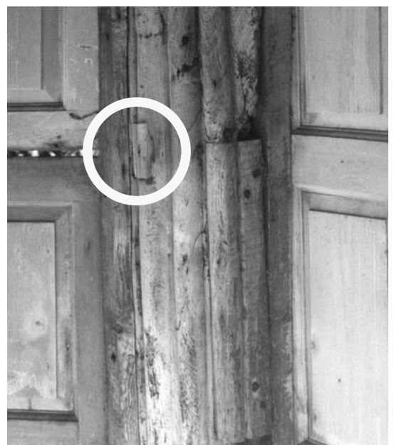
Post 3 showing the mortice (see figure 3).
