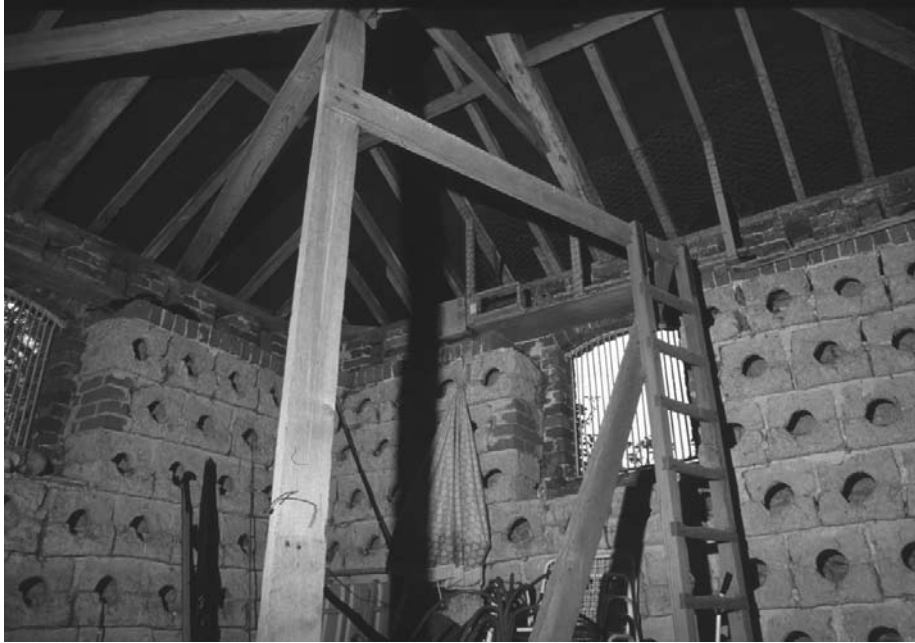
The interior of an early 19th century dovecote at Thickthorn Hall. Note the revolving ladder, and nest-holes of clay lump specially moulded to shape.
