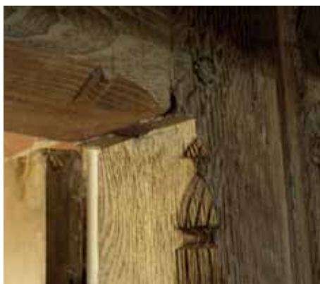
Doorframe detail showing the bar-shield-and-notch chamfer-stops
