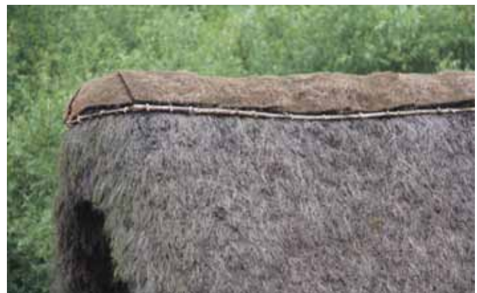
Turf along the ridge as a retainer, above thatch made of heather
