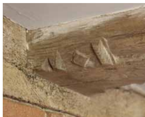
Sunk-quadrant chamfer with bar-diamond-and-pyramid chamfer-stop photos this page: Michael brown
