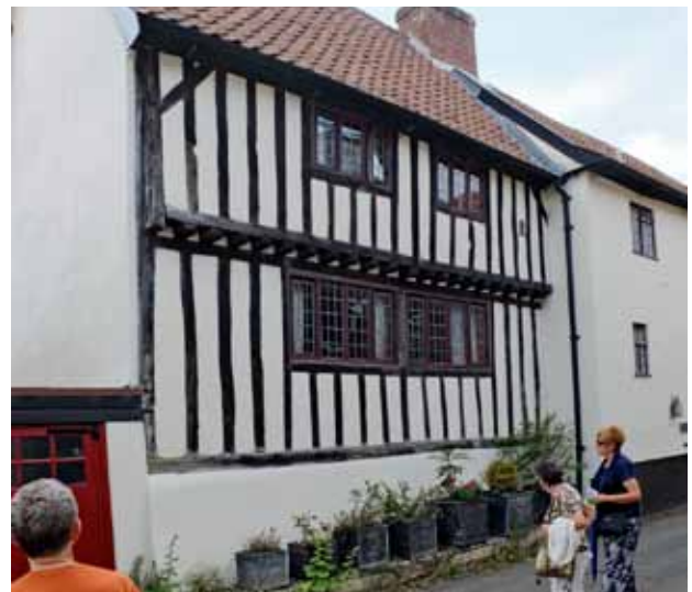
The Cardinal's Hat in Back Street with its hewn jetty posts (Richard Ball)
