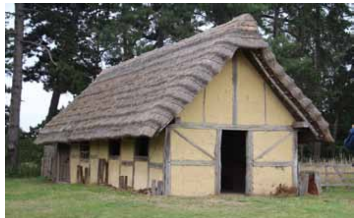
One of the hall-type buildings with thatch anchored along its length with a combination of willow withies and straw rope
