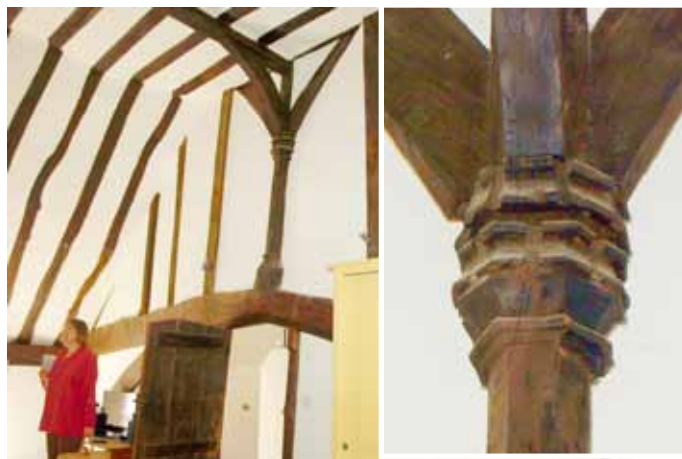
The principal crown post in situ and the brattished head in detail
