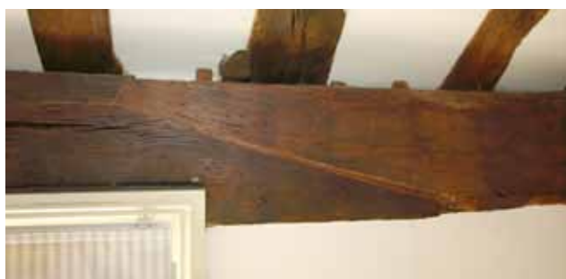
Splayed and undersquinted scarf joint
