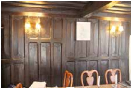
The screen adjacent to the crosspassage, seen from the hall, with its elaborately carved panels and a doorway, blocked to match the panelling
