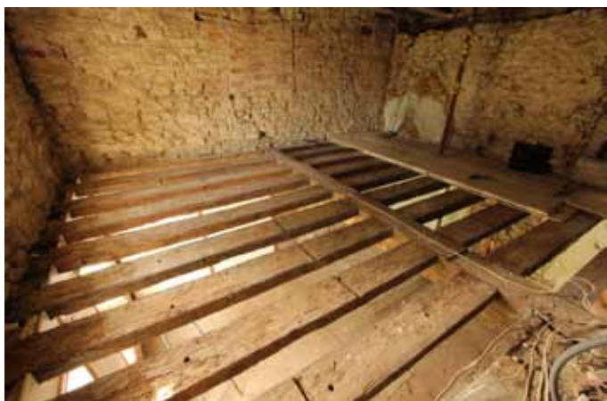
Twelfth-century timbers reused as sixteenth-century floor joists
