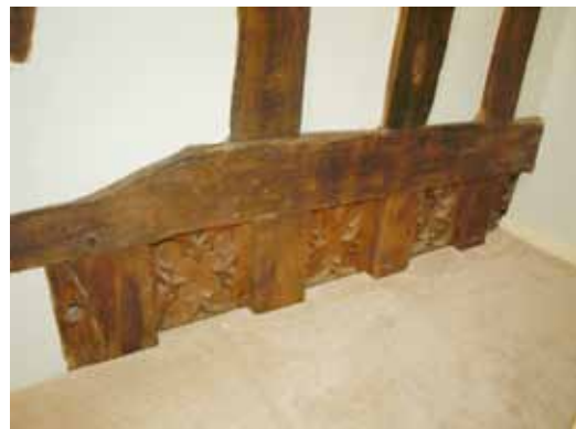
Quatrefoil tracery above the service doors - see also recon- structed view from the hall, next page
