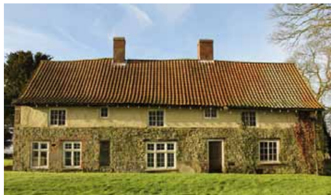
Lincoln Lane Farmhouse, eastern elevation
