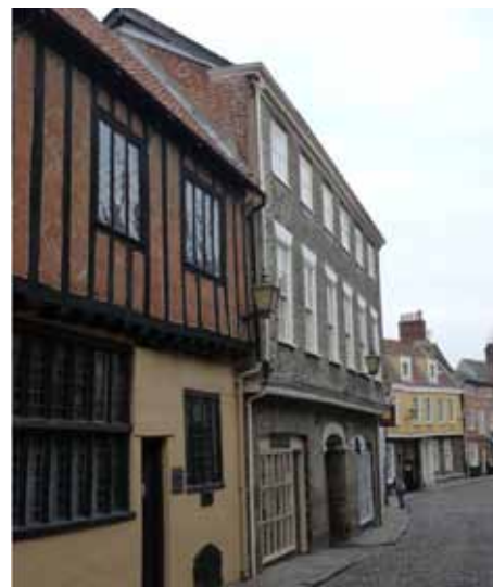
28-30 Elm Hill - bricked-up, symmetrical, front, but still displaying the earlier jetty
