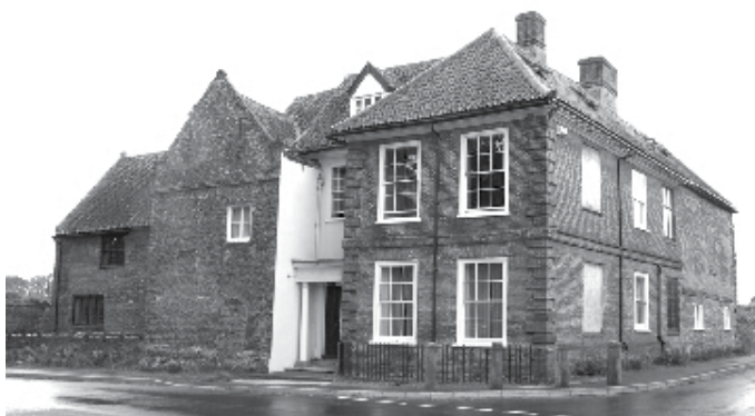
Fig. 4a Manor House, Worstead: south front and east side elevations. The oldest part of the house is thought to be to the left of the picture. The weavers' loft/eighteenth century saloon to the right in the area with no windows on the first floor.
