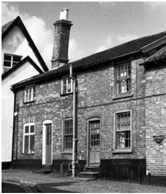
Fig. 3 Nos. 33 and 35 Damgate
