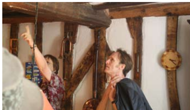
Fig. 8 Discussions on diagonal bracing in The Old Rectory.
