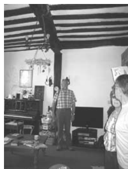
(b) high ceilinged ground floor room with moulded axial joist.
