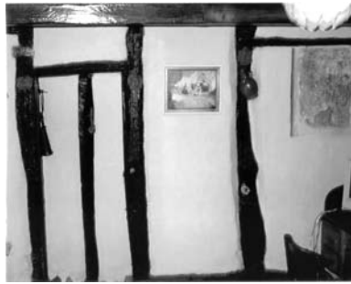
Fig. 4 No. 33 Damgate: stud wall.
