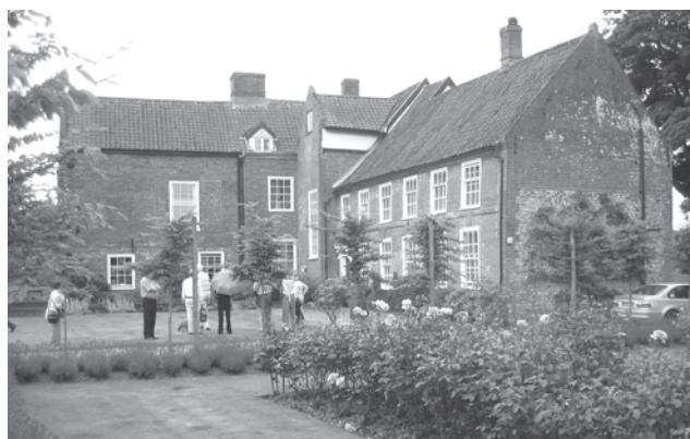
Fig. 4b Manor House, Worstead: north garden and west garden elevations. The weavers' loft/eighteenth century saloon is to the left; the oldest part is behind the brick facade.
