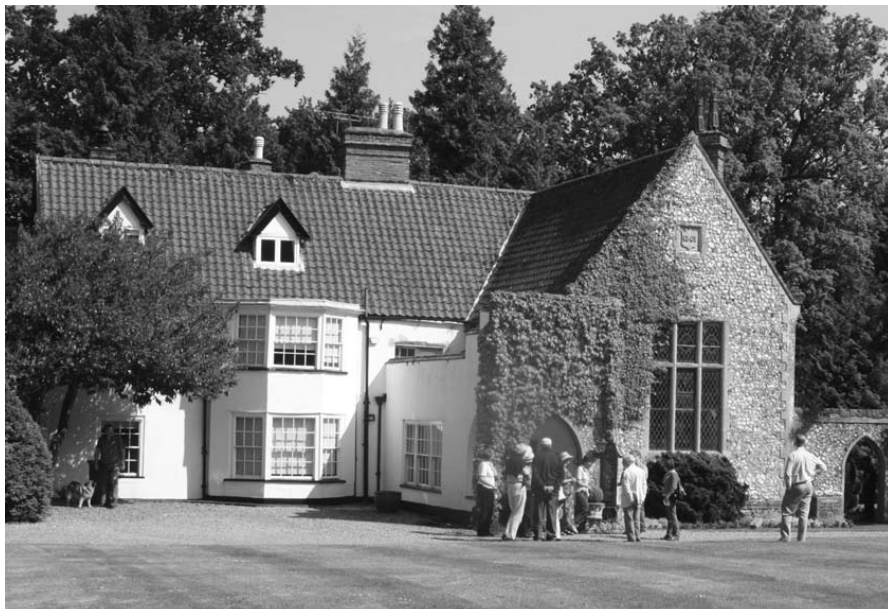
Fig. 7 The Victorian Sunday School wing in the flint building.
