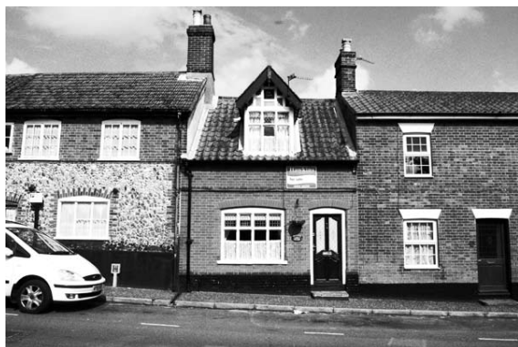
Fig. 6 Nos 39 and 41 Damgate: flint facade which is probably the height of the original roof line.
