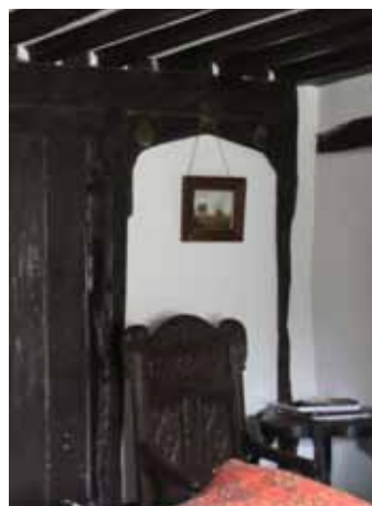
The original cross-passage doorway in the back wall
