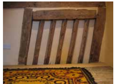
the racking of the upstairs-window mullions
