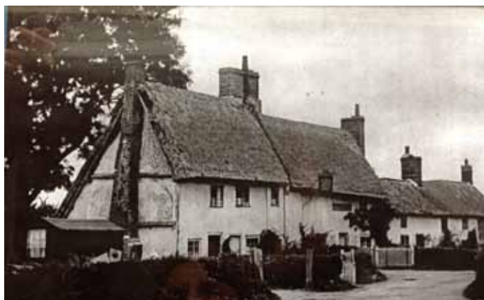
The Old Nag's Head, probably in the 1870s. The right-hand side used as a pub (with its hanging sign), and the left-hand side as two cottages (note the two front doors). This meant that the room to the left of the chimney stacks was divided into two, hence the need for the additional gable-end stack at the near end, since demolished. The stack at the other end belongs to the neighbouring cottage
