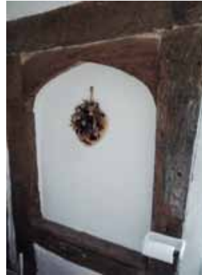
above left: the early shop window at the west end from the inside above right: the window as it exists now, illustrating the settling of the western end of the frame
