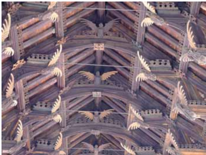
Detail of the roof at St Wendreda's, March (photo: Rob Walker)
