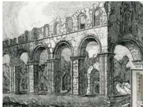
above: The Infirmary during demolition
