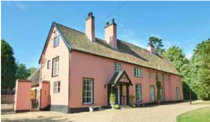
The Old Rectory, Long Stratton
