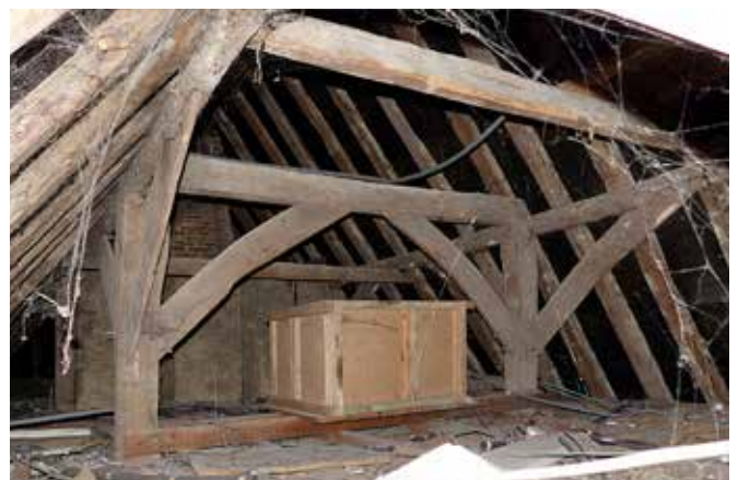
One of the substantial queen-post roof trusses
