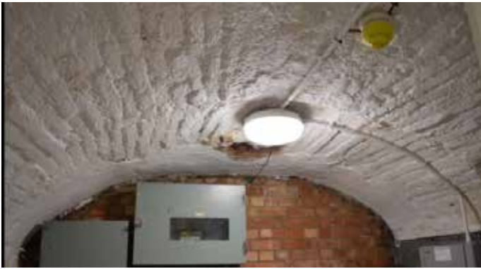
A barrel vault at 21 Bedford Street
