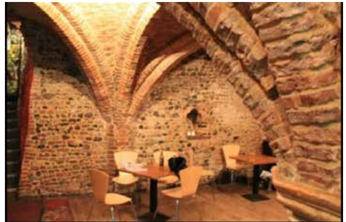
Central pillar and ribbed vaulting at Bedfords, enlarging the space available
