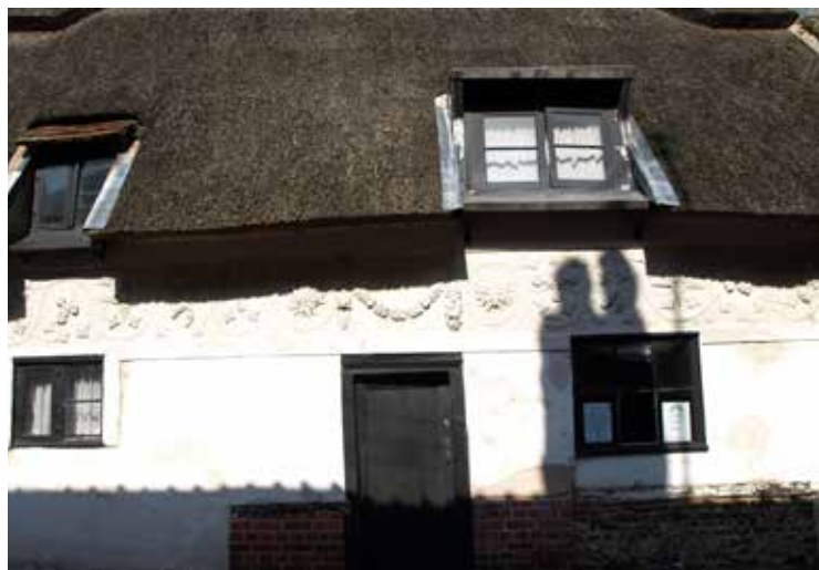
The elaborate pargetting on the front wall
