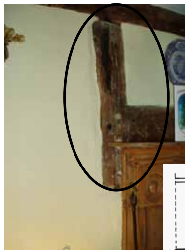
left and below: Timber-framed chimney at Riverside Farm, Fornsett St Mary - dendro-dated to 1645
