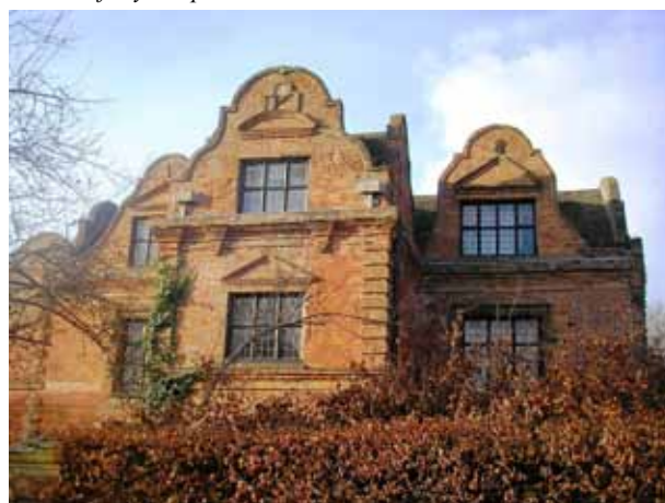
Perhaps the earliest curvilinear gable in Norfolk - at 54, Bracondale - dated 1578, with both round and ogee gables, in English bond. Wall anchors show 1578, although reputedly built for Anne Kempe in 1620, and the rainwater hoppers show 1656 with the initials on one of R over AE and on the other R over ME - presumably a later addition by a new owner.
