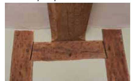
above: Principal joist support at Lundy Green Farm, Hempnall, notched, tenoned and pegged left: support of the axial joist also on the frame, rather than jointed into a post, at Fairbanks House
