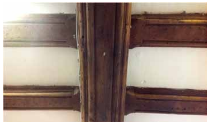
below: the inserted roll- moulded floor joists
