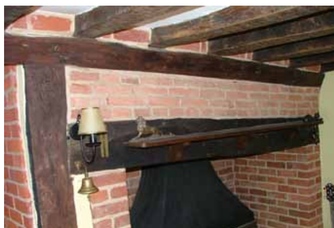
above: Timber-framed chimney (now bricked in) at 44 Norwich Road, Tacolneston
