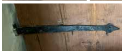
Two of the retained plank doors and one of the hand-made strap hinges
