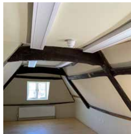
above: the typically seventeenth-century roof construction
