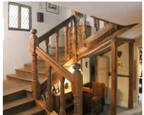
above: inserted seventeenth-century oak staircase
