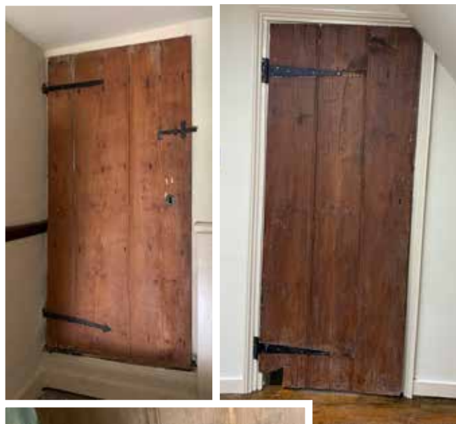
Two of the retained plank doors and one of the hand-made strap hinges
