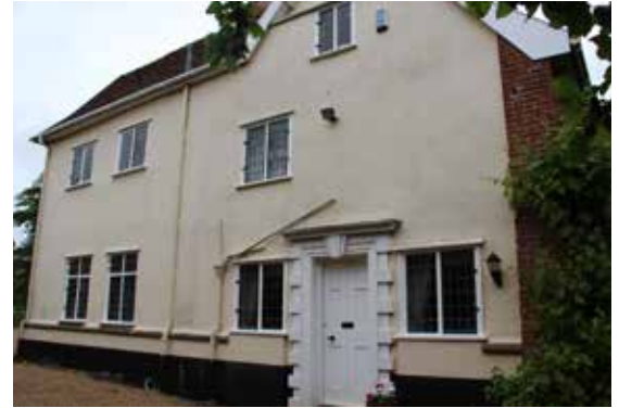
phases 1 and 2? from the south-west
