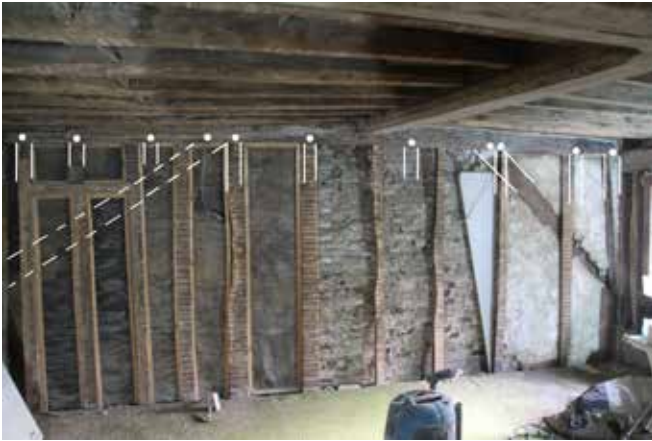
hall chamber east wall showing the lack of a mid-rail and the inserted doorway with different stud spacings from the originals.
