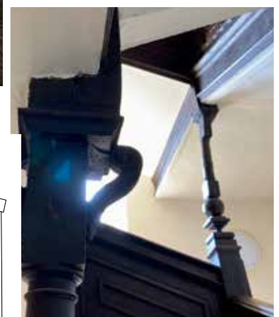
The magnificent staircase showing some of the "pillars" needed to reinforce the structure
