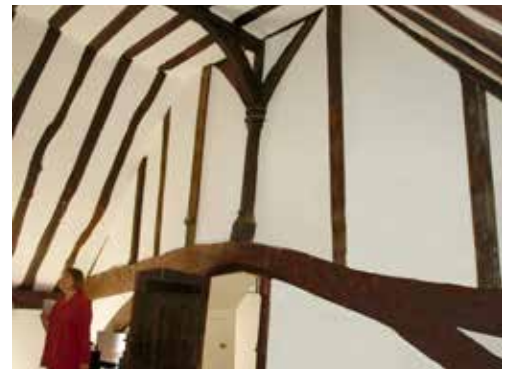
Below: A similar roof at 3-5 Castle Street, Thetford (also awaiting dendro)
