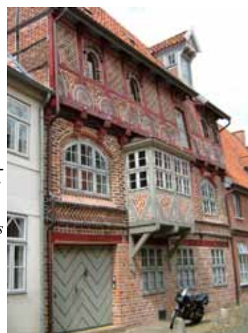
right Brick-built ground floor, jettied upper storeys in Luneburg. Moulded brickwork and carved brackets with elaborate paint schemes
