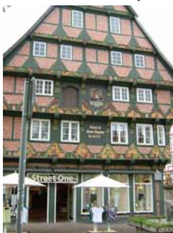
left Timber-framed gables in Celle with multiple jetties and triangular braces. Shop windows disappeared
