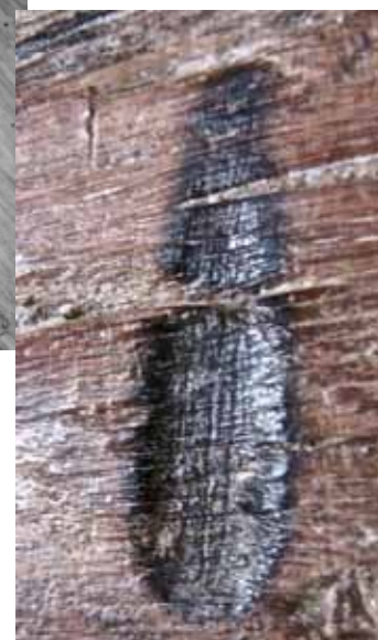
Figure 3. Evidence of removal of charcoal crust by scraping, leaving scratch marks (Oxfordshire)
