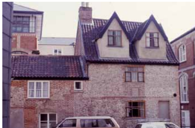
Restoration of 17th century weavers cottages - 1986
