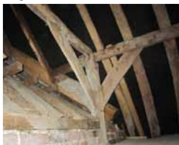
The queenpost truss that confirms that the crosswing (the roof of which is seen to the left) is later than the original build
