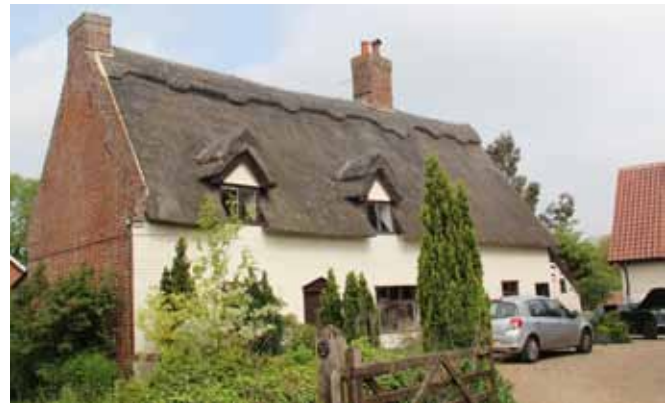
The Chestnuts - much the same as when it was built, in around 1600, apart from the additional brick gable and stack on the left-hand side
