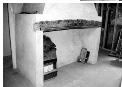
First floor: Fireplace—west facing (towards Market Place) stack top cut off
