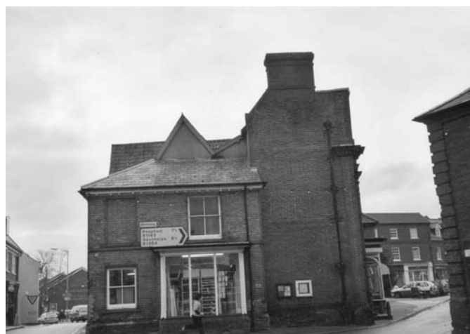
An example of later Market Place infill showing at least three distinctive periods of construction.
