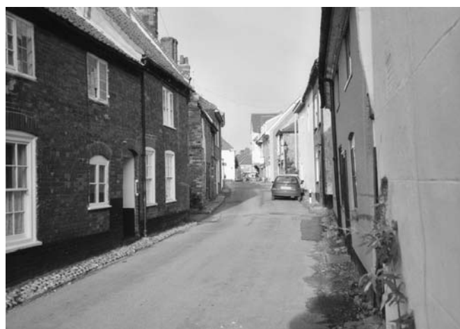
Hungate Street. The Medieval approach to Aylsham from Norwich. Probably several early Sixteenth Century properties survive.
