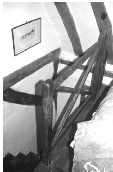
Beech Cottage: simple Georgian stair rail
