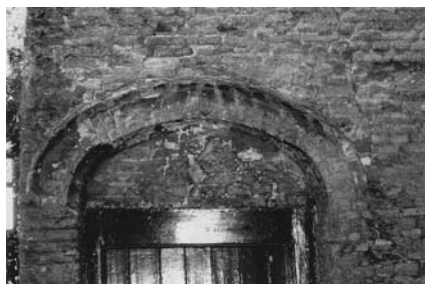
Sandwich, Kent: An Anglo-Flemish house of 1603, with a similar plan and wall-anchors to the Yarmouth row houses. Both were the result of cultural links through migration, but Sandwich has Flemish gothic brick details and Yarmouth Flemish structural carpentry.
