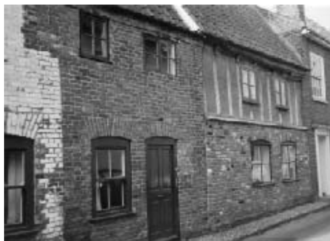
No 18 Hungate Street. Parts of this survival date from c 1500, including an intact oak mullioned window.
