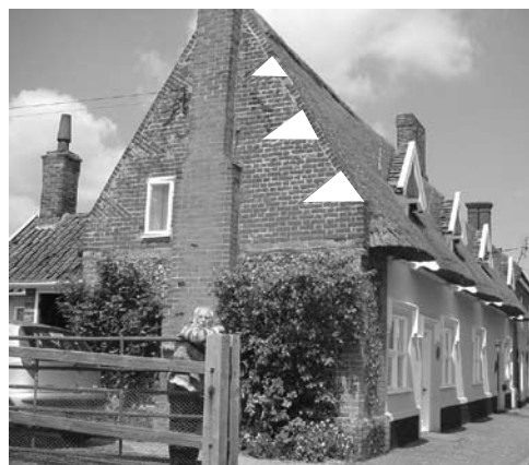
A Norfolk eighteenth century, clay lump cottage (and very proud owner) in Church Street, Carbrooke. Note the plinth and the tumbling-in (see p.2).
