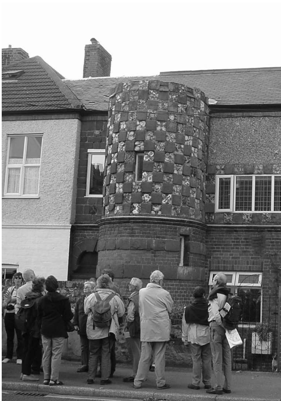
New Hunstanton in September 2004. This flint chequerwork tower has visual links to the building of the Hall in Old Hunstanton and the Scottish Arts and Crafts Movement (see pages 6 and 7).
