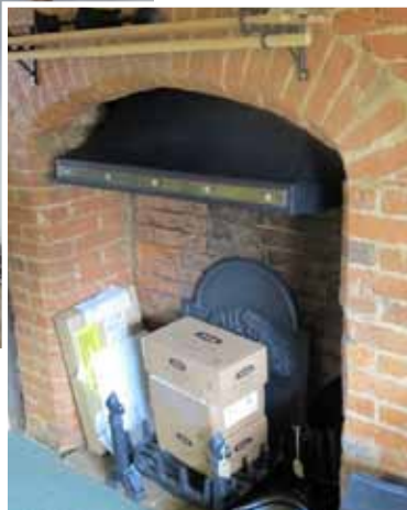
Brick fireplace with carefully-cut chamfers
