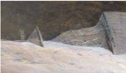
Lamb's-tongue stop and a nick on the principal joist
