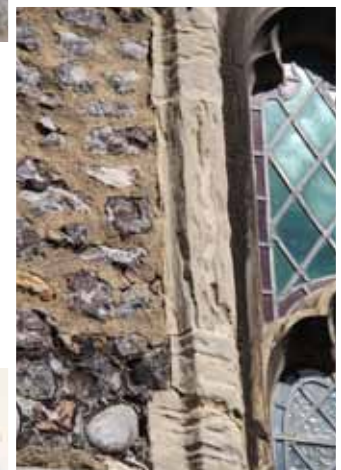
Two samples of Clipsham stone, showing how different they can be - one fine and one coarse grained and different colours (Ian Hinton)
