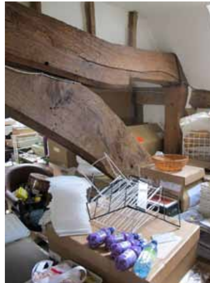
above: roll-moulded principal joist with elaborate moulding on the common joists as well
