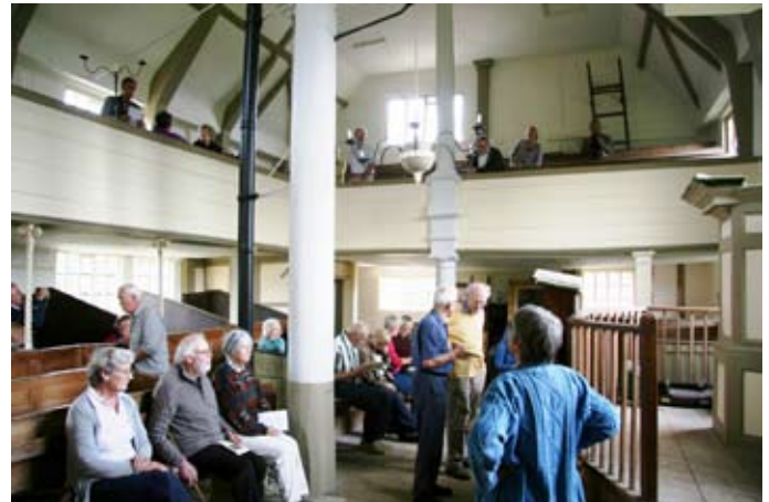
The galleries in Walpole Old Chapel and the cast iron columns holding the roof up. (See Anthony Rossi's article on page 4).
