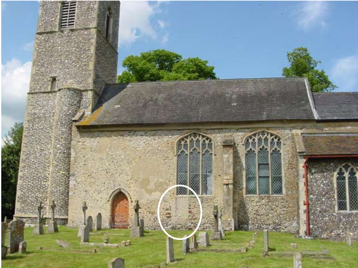
Braydeston Church: this photo shows the original door which was blocked up when the church was extended westwards. The tower may have been added as part of this exercise.
