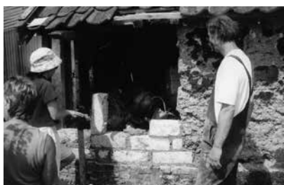
Making clay lump in 2001, guided throughout by Richard Hyde - Diana and ? making clay lump
