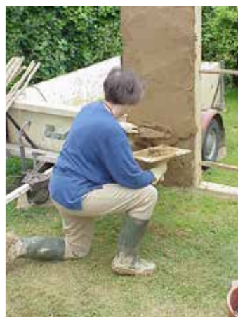
? rendering the completed daub
