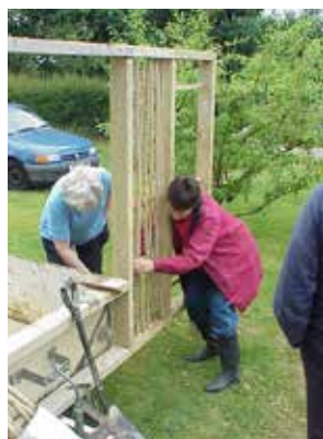
Wattle and daub in 2001 - ? and Richard mixing the daub and Carol and ? beginning the application
