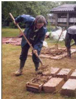
Making clay lump in 2001, guided throughout by Richard Hyde - Diana and ? making clay lump
