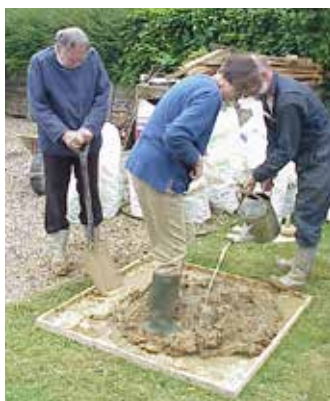
Wattle and daub in 2001 - ? and Richard mixing the daub and Carol and ? beginning the application
