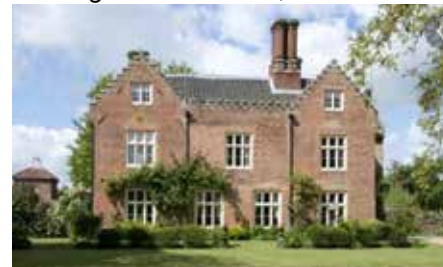
Old Hall, East Tuddenham 2004
