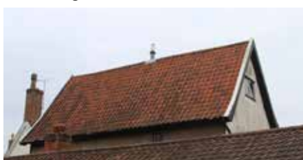
Diss Iron Works, 2016
