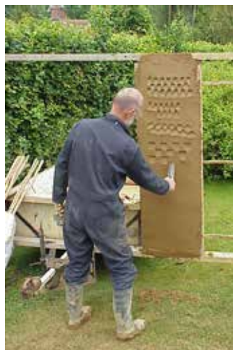
Richard doing some elementary pargetting on the completed daub.
