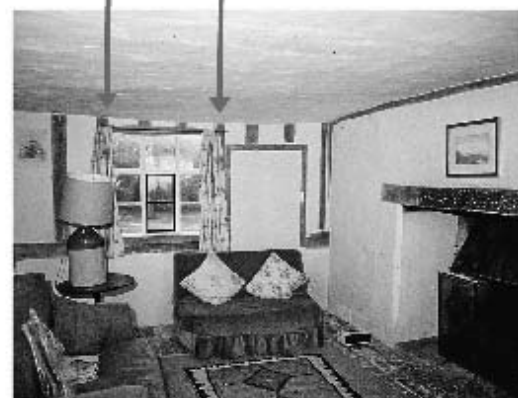
Fig 2. Rear wall of parlour (below) and parlour chamber (above). The head of door inserted before the parlour was raised is just above the floor on the right on the first floor
