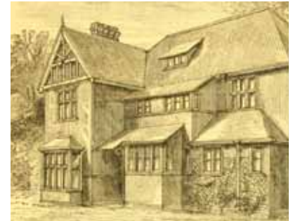
No 408: The largest corrugated-iron-clad house in the 1888 catalogue
