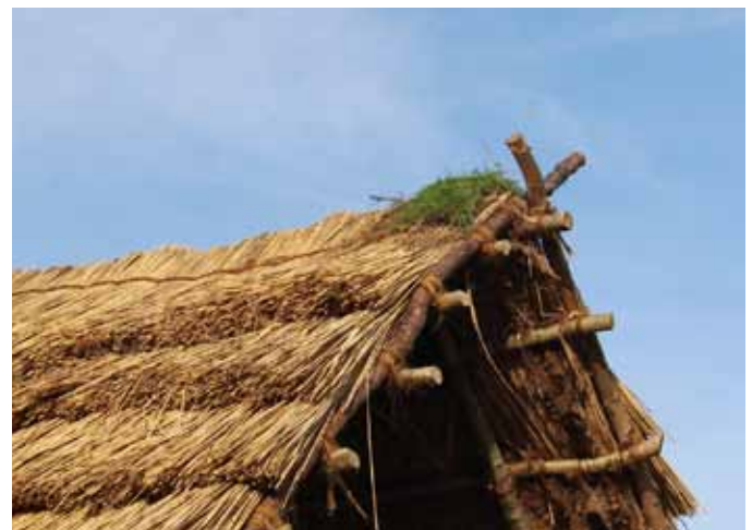
above: Layered thatching on the reconstructed Stone-Age longhouse below: The first turf covering the rot-prone first line of rope which stitches down the thatch (photos: Ian Hinton)
