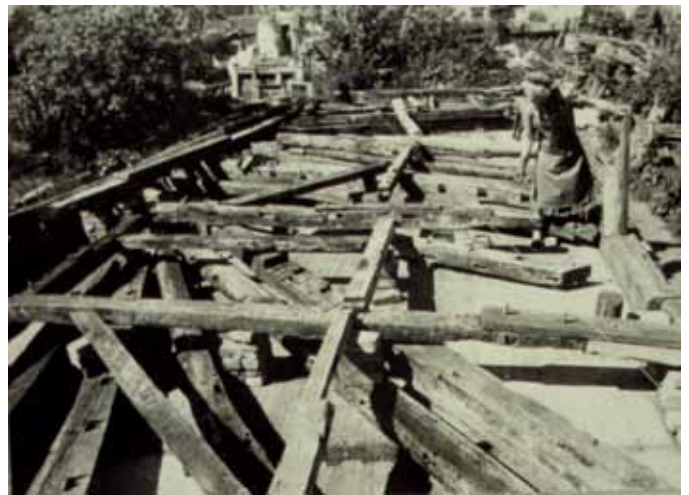
Some of the many photographs documenting the prolonged process of sorting and re-assembling a complex timber-framed hall house
