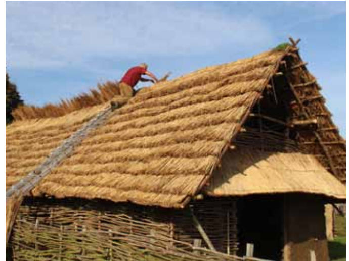
above: Layered thatching on the reconstructed Stone-Age longhouse below: The first turf covering the rot-prone first line of rope which stitches down the thatch (photos: Ian Hinton)
