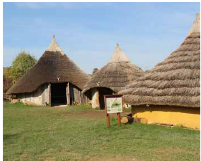
Three of the Iron-Age round houses showing the earlier smooth thatch on the left and later layered thatch on the right
