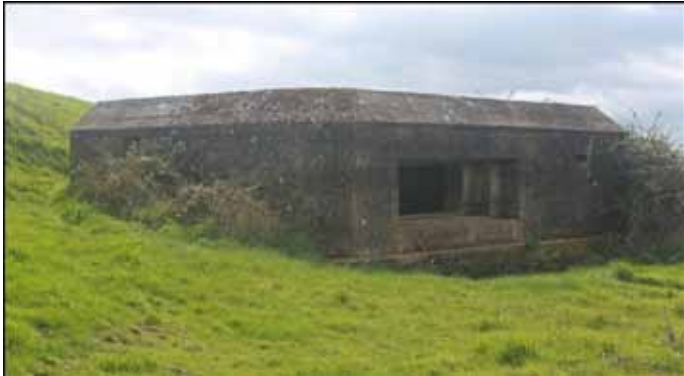
An anti-tank pillbox at Heacham. The nearby beach was considered suitable for landing tanks and so was provisioned with suitable defences. In contrast to many infantry pillboxes, the workmanship of this structure is high.
