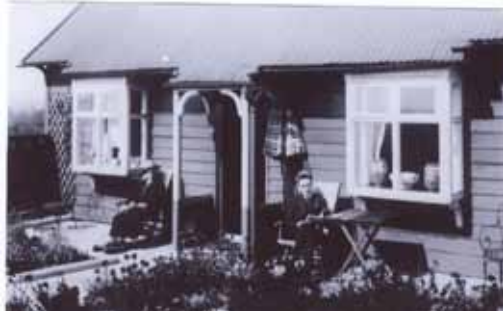
Rookery Cottage: timber clad, built in 1891
