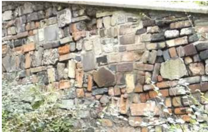
The boundary retaining wall, including robbed freestone
