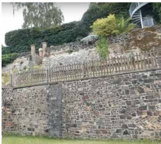
Two of the terracing walls, one above the other, supporting the chalk escarpment
