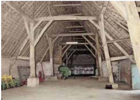
Plate 3 Hall Farm Barn looking east with truss 3 in the foreground
