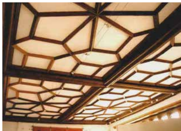
Below: The ground-floor parlour decorative battened timber ceiling
