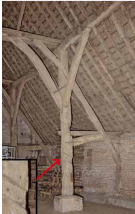
Plate 4 South arcade post of truss 6 with lower passing trench highlighted
