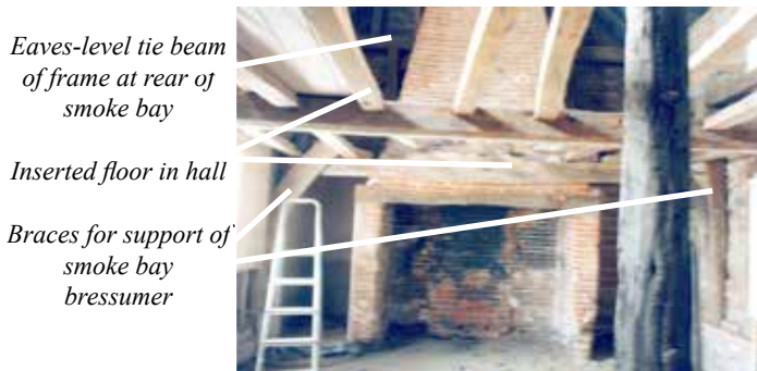
Photo 2 The hall and smoke bay with inserted brick stack
