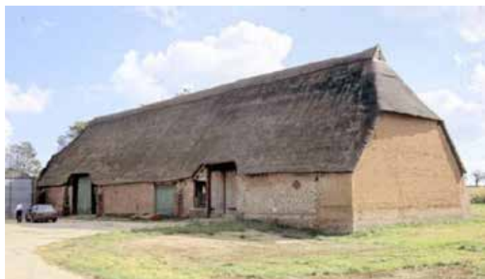
Plate 1 Hall Farm Barn north front
