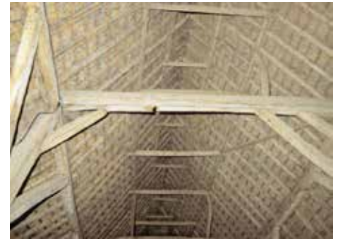
Plate 5 Hall Farm Barn roof looking east from truss 5
