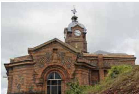
Eye Town Hall from the south, showing the use of red and yellow bricks
