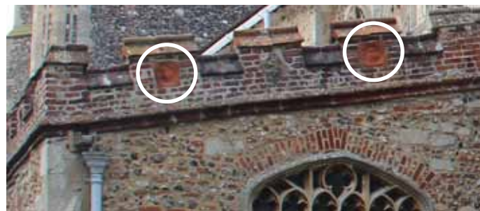
Terracotta panels set into the chapel battlements
