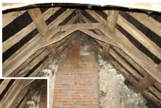
34 High St.- above - the arched braces and collar left - the cranked principal rafter. photos: Michael Brown
