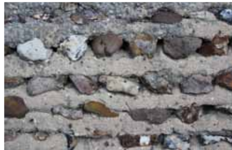
Original Norman flintwork in the nave wall at St Mary, Thornham Parva
