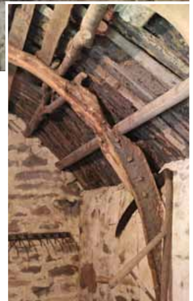
Above - manufactured "crucks" and multiple "purlins"
