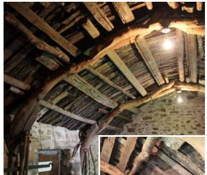
Above - manufactured "crucks" and multiple "purlins"
