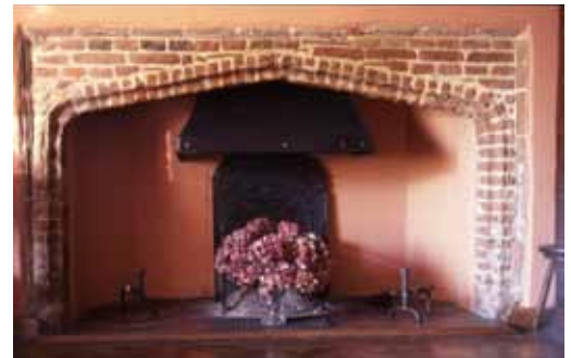
Brick hearth in the parlour with elaborately cut bricks
