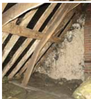
34 High St.- above - the arched braces and collar left - the cranked principal rafter. photos: Michael Brown
