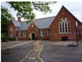
Fig. 5: H-plan school at Blofield, built in 1877 by a school board still retains the traditional gothic look.
