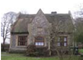
Fig. 1: The picturesque ‘cottage style’ school built in 1834 at Witton by Lady Wodehouse.
