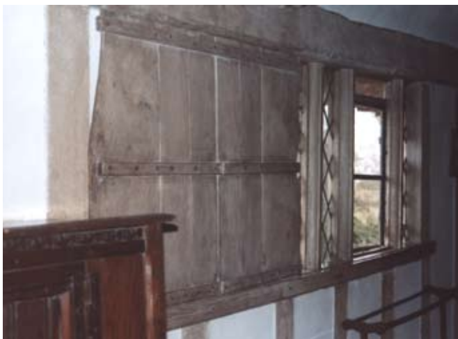
Photo 2 Shutters in place Manor Farm, Pulham Market.
