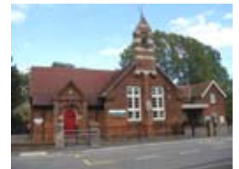
Fig. 4: The Board school at Beeston, near Mileham incorporates a variety of architectural styles.
