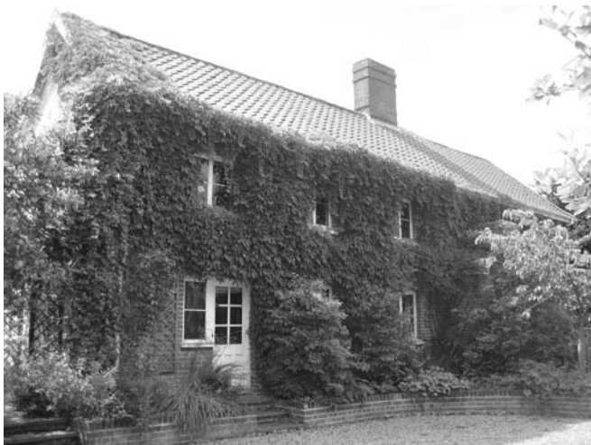
Bridge Green Farm, Burston: who would have thought this brick and tile, Victorian-looking house would hold a queen post roof. One give-away is the location of the stack which divides the roof into one third and two thirds.
