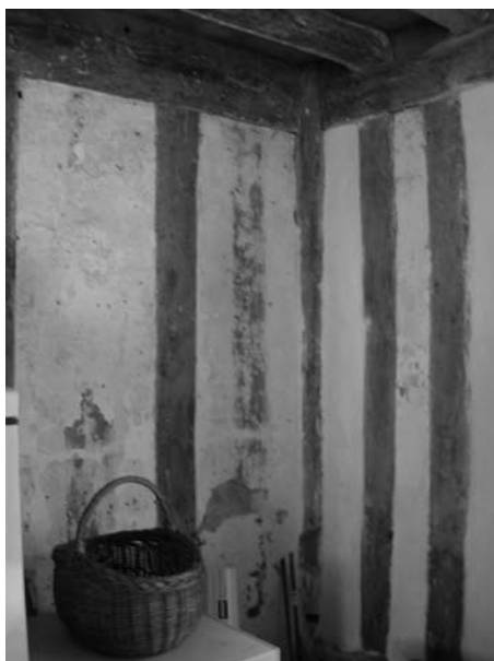
Some studs on the ground floor are painted onto the plaster as opposed to being genuine timber studs. The tops of them have been decorated with wall paintings to give the impression that they have capitals.
