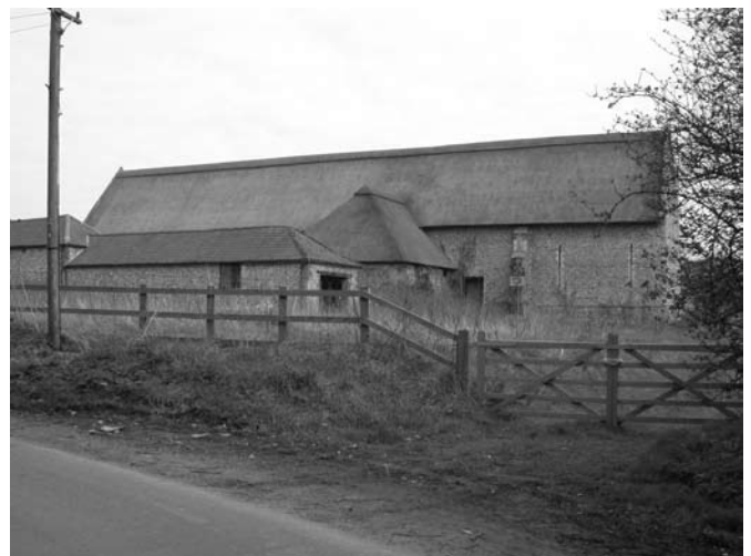
Paston Barns in their restored state.
