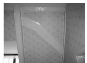
Cranked brace (see also Gissing p.10)
