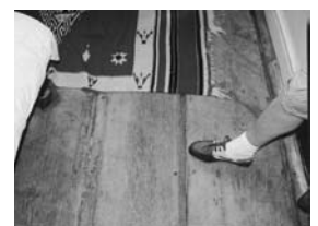
Broad oak floor boards of original build
