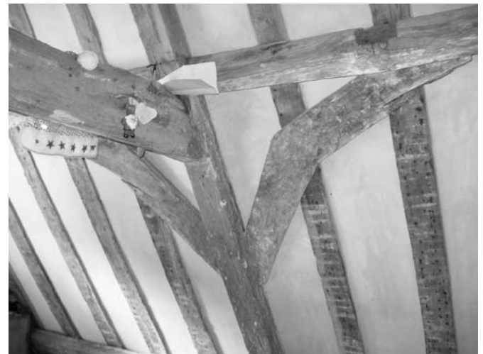
'Cranked' windbraces (see also Rainthorpe Hall p12) which still bear traces of raddle.
