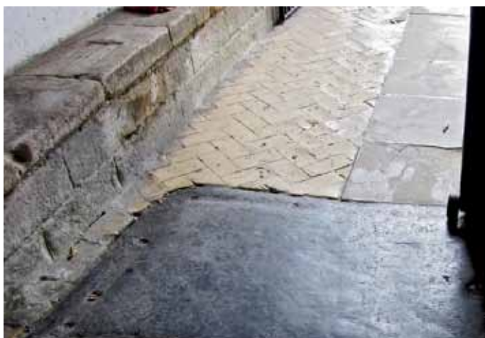
Part of the ledger slab which dominates the porch floor at Terrington St Clement, showing the holes for the fixing of the original brasswork (photo Richard Ball)
