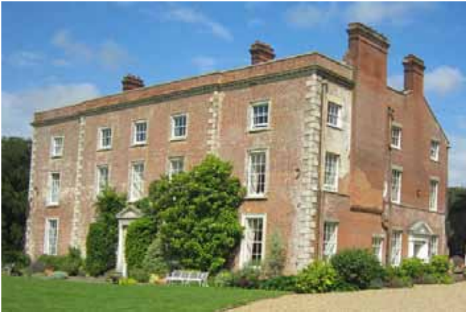
Bayfield Hall's southern elevation (photo Rosemary Forrest)
