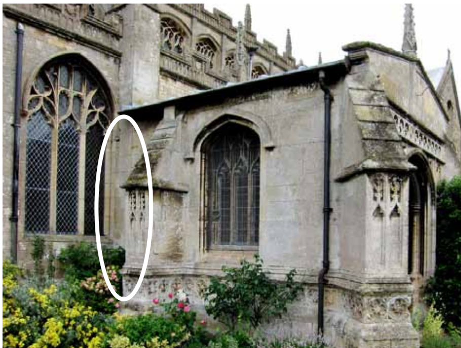
Terrington St Clement porch, built after the aisle - demonstrated by the butt-joint with the buttress (joint highlighted) (photo Richard Ball)
