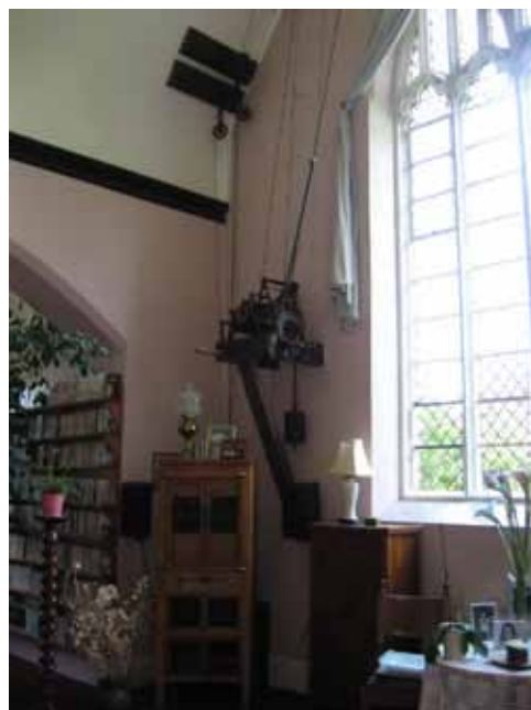
The 1892 clock mechanism at Hardingham. It is easy to understand why it is too loud to have it running
