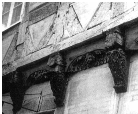
D - elaborate carved jetty brackets
