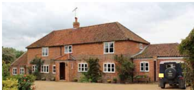
Meadow House; farmhouse --► cottages --► back to single house (photo Maggy Chatterley)
