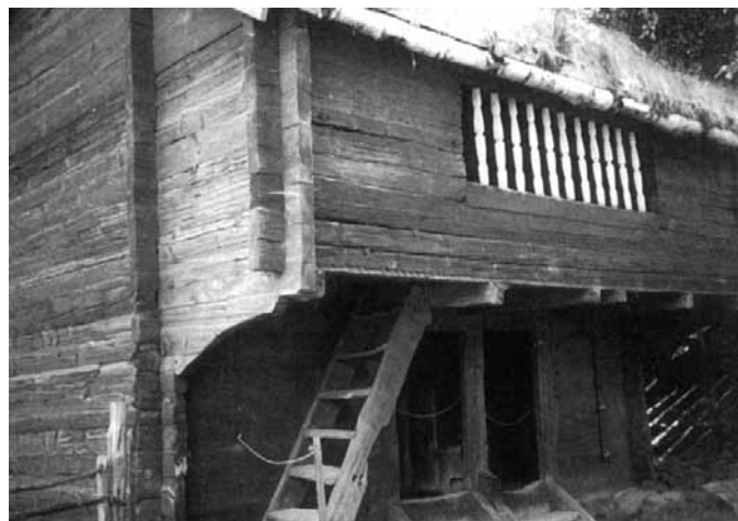
A - ‘Log cabin’ corner construction
