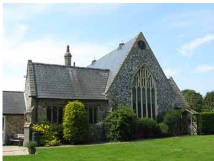
Hardingham School, now closed and converted into a private house (photos Susanna Wade-Martins)
