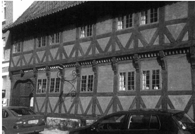
C - urban jettying, showing the 'panel-filling' windows
