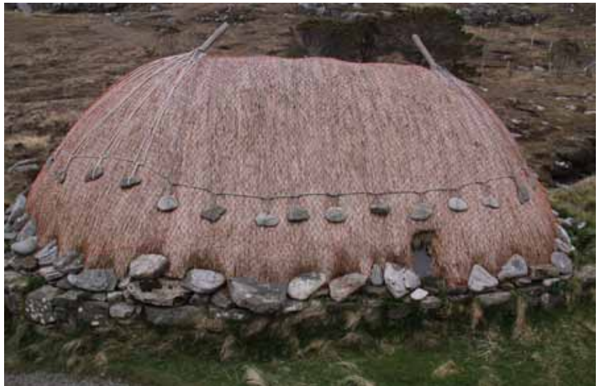
above: The mill at Shawbost, with Hebridean double hipped ends with "crow posts" and roped-together stones
