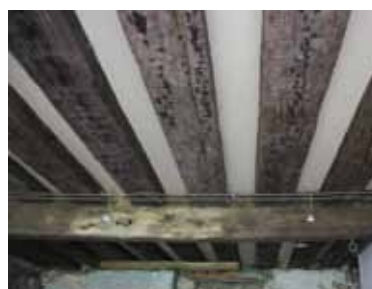
Photos: Ian Hinton left: The substantial joists from the Priory cloister, brought in as part of the seventeenth- century changes to the house
