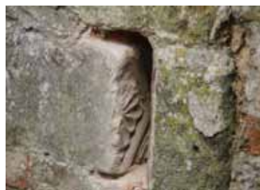
left: One of the reused stones from the monastery, thought to be one of the double capitals from the cloister. Here the carved face was hidden as the smooth worked face was required for the outer surface of the wall
