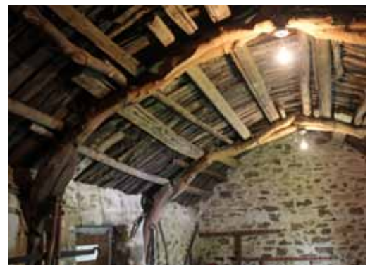
Caithness - manufactured crucks and multiple "purlins"
