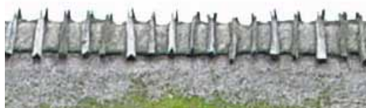
Danish crows' beaks retaining the thatch (photo: Robin Forrest)
