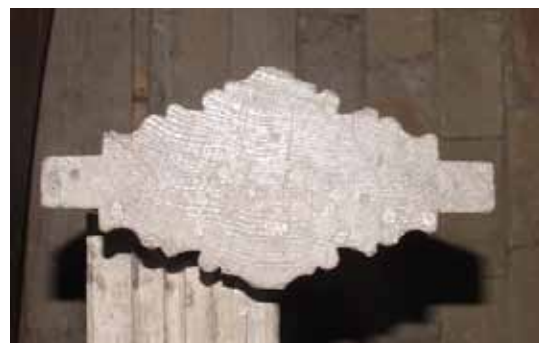
left: The complex cross-section of the sawn-through screen post
