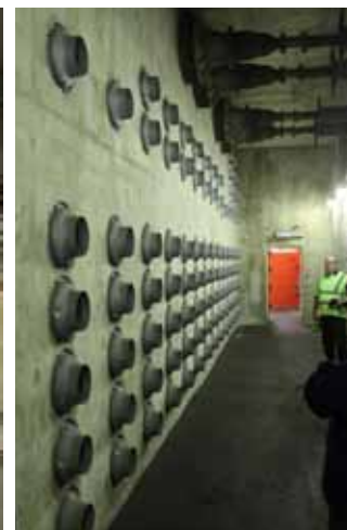
some of the pressure-absorbing mechanisms in the event of a nuclear blast
