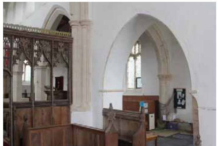
The apparently 11th or 12th century arch into what may have been the northern transept
