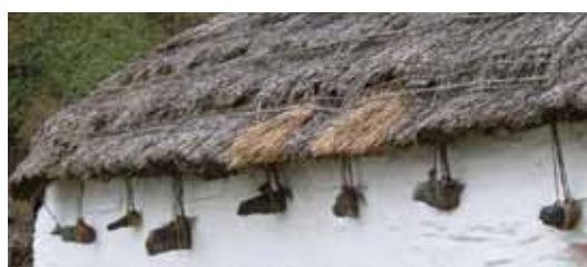
Isle of Man - projecting stone anchors
