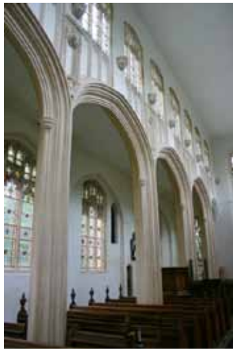
The spectacular nave arcade moulding and the extended clerestory mullions providing a unified scheme
