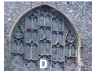
Shouldered ogee arches of the fifteenth-century rebuilding in the north aisle
