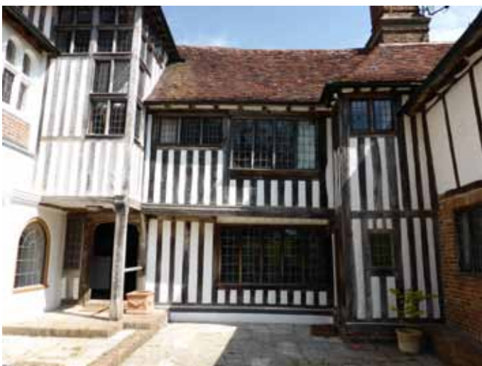
Frensham's south façade, showing part of the sixteenth-century continuous-jetty wing in the centre, and the side of part of the fifteenth-century building on the right.
