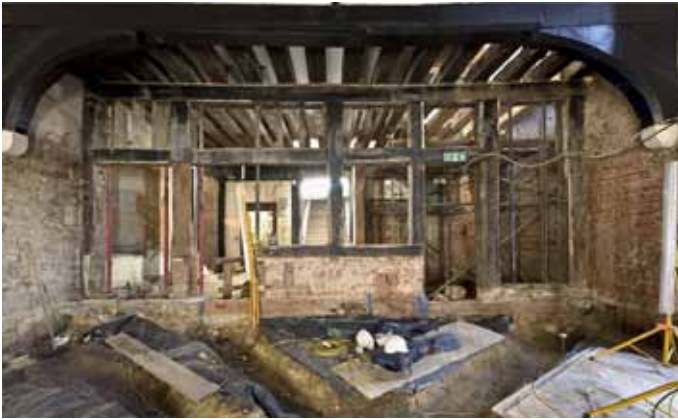
above: The kitchen west wall showing exposed timbers of 1382-3 serving hatches, modified in 1882.
