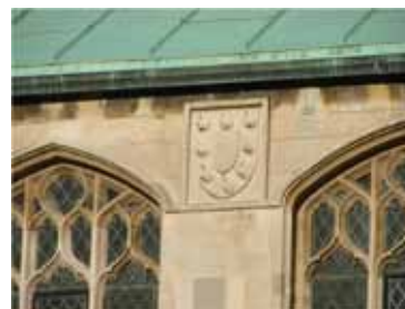
The Erpingham Arms plaque between each clerestorey window
