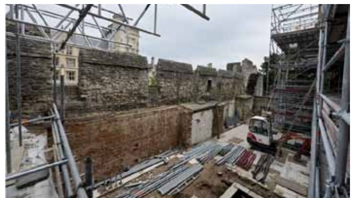
City wall from the buttery, following demolition of the 1882 ancillary buildings.
