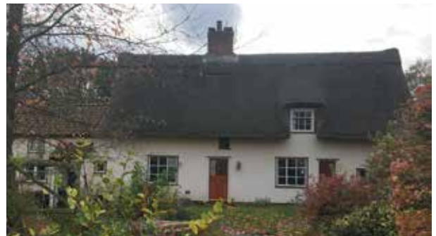
The Nuttery from the front (above) and rear (below during restoration)
