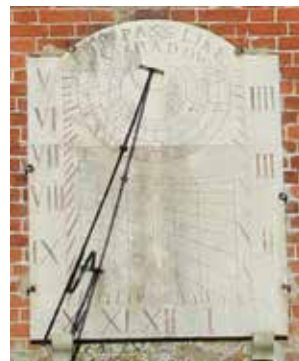
Grundisburgh (Suffolk) declining gnomon to cater for the church alignment of 68°
