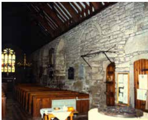
One of the many churches that had their wall plaster stripped under the guise of mediaeval authenticity
