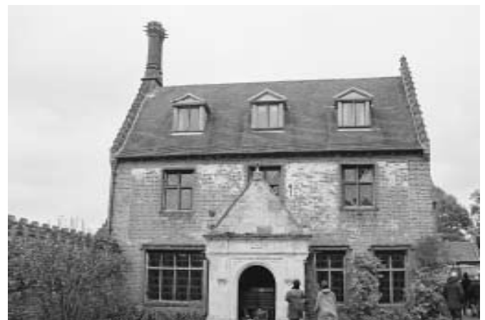
This is said to be the earliest build and was originally timber-framed. Two bays on the garden wall side are missing; the remaining range has wrap-around brick gables, and there is an impressive ashlar-faced porch with a date stone of 1574.
