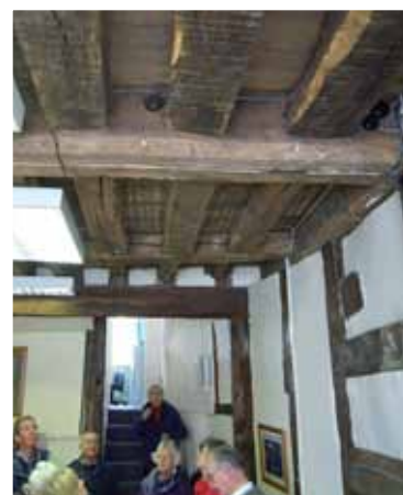
Figure 2 - Cavendish House, ground floor joists (photos John Dean)
