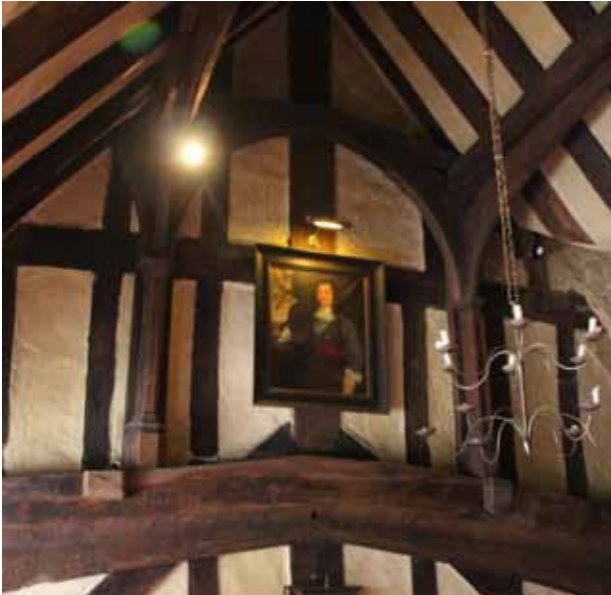
figure 5 - White Hart queenpost roof (photo Ian Hinton)
