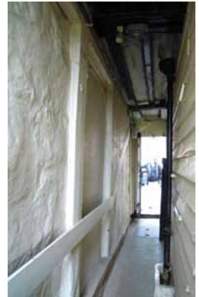
figure 8 - cross passage and service doors (photo John Dean)
