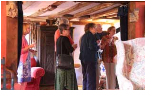
Investigating the doorway for the stair to the service chamber (left)
