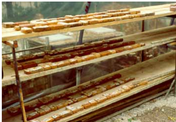
Storing the bricks between dismantling and re-erection
