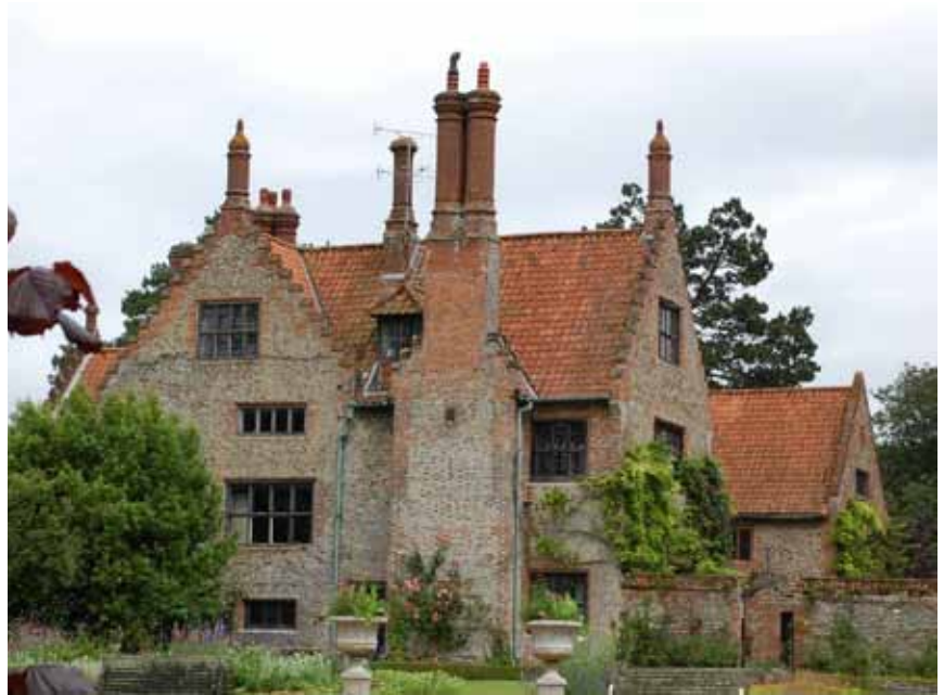
Hindringham house from the west, emphasising the stepped gables (photo Billy Jones)
