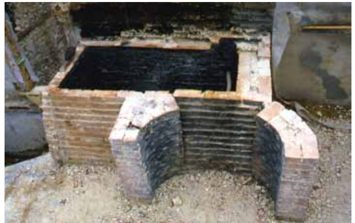
Below - The hearth/chimney during dismantling
