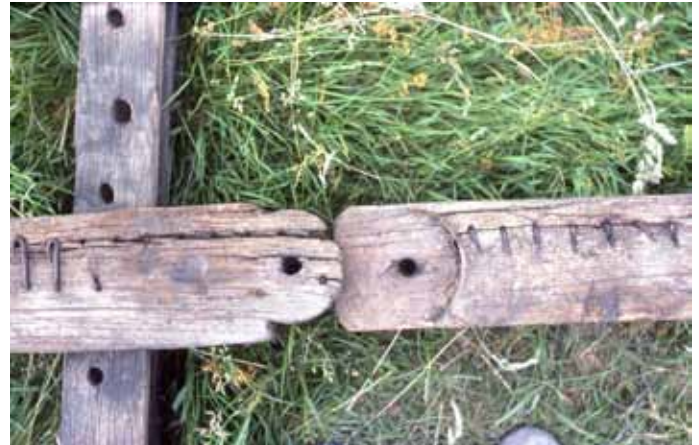
Elland Old Hall: timbers of a tenterframe that had been re-used as floor joists.
