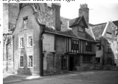
One of the smaller houses (No 29) on the right, with a C19 brick range added to a C17 flint building
