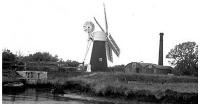
Polkey's Mill and steam engine house
