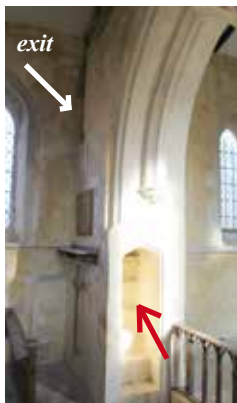
right: Internal stair built within the structure at Coston
