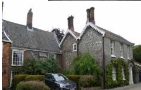
Baret's House (No 69) built in 1549 with a rubble ground floor and timber jettied upper storey - with a later brick gable. (photo: Plunkett collection)
