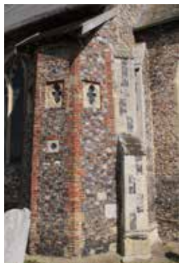
right: Internal stair built within the structure at Coston
