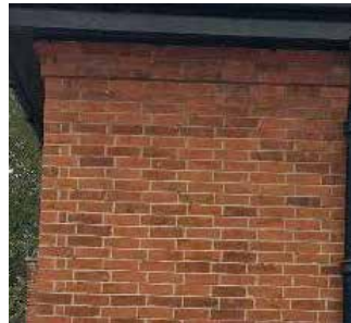
above: the oddly-spaced, stretcher-only, brick bonding left: the reused lavabo, stoup or piscina in the clerestory embrasure
