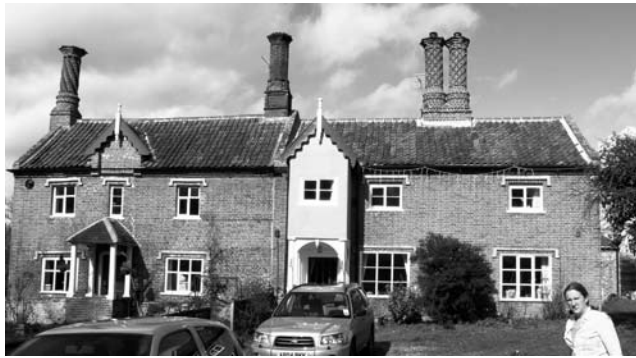
Woodyard and Estate Yard Cottages
