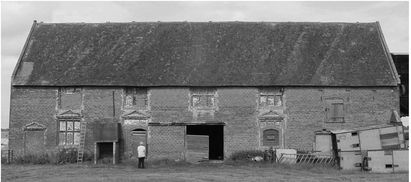
West front of the barn
