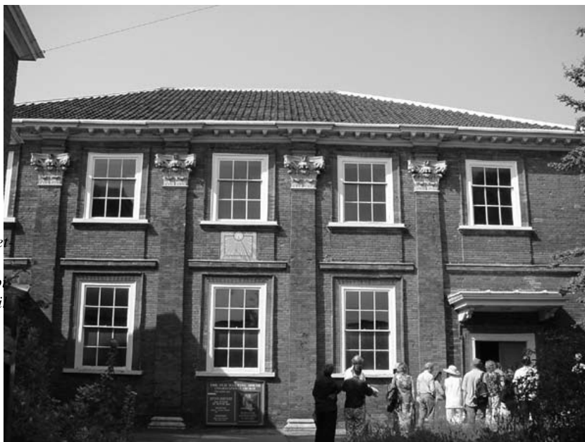
The Old Meet- ing House: Corinthian pi- lasters, detail and interior
