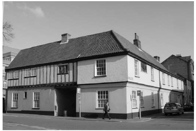
Muspole Street, Norwich: timber framing, medieval mullion windows, and modernising mathematical tiles. (Photo: B Fenner)
