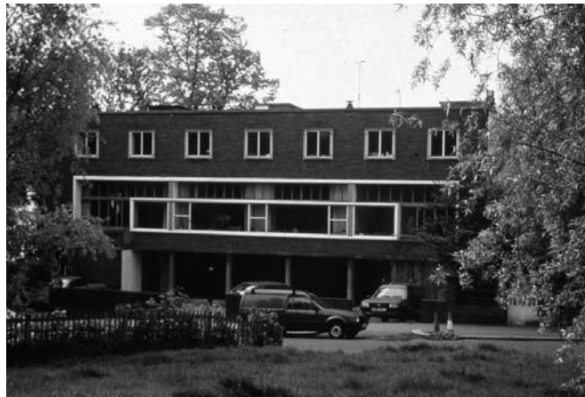
Close view of front elevation showing structural concrete pillars and photobolic screen (National Trust)
