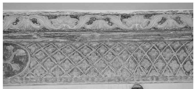
Irregular quilting: The diamond shapes are almost square on the left and very elongated on the right
