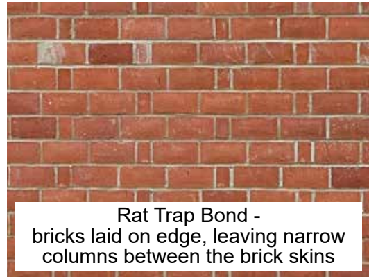
Un-named Bond - two headers one stretcher (Irstead)
