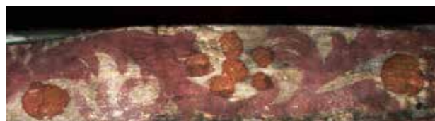
Above: Painting on one of the common joists
