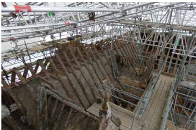
Figure 1 - The ongoing roof work
