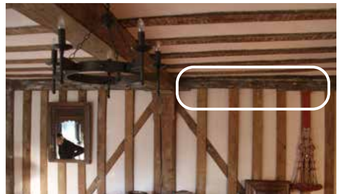
The ground-floor north wall of the crosswing, showing the 1960s replacement studs, neatly pegged into the mid rail on the left of the storey post, but to the right is evidence for a window and shutter slide in the soffit of the rail
