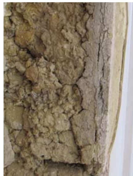
Figure 2 right: clay lump with plaster skin.
