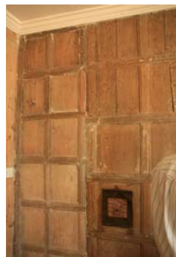
Old Hall farm House, Foulsham: reused pine panelling an upside down taper burn – an indication that the panelling is reused.
