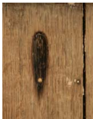
Old Hall farm House, Foulsham: reused pine panelling an upside down taper burn – an indication that the panelling is reused.
