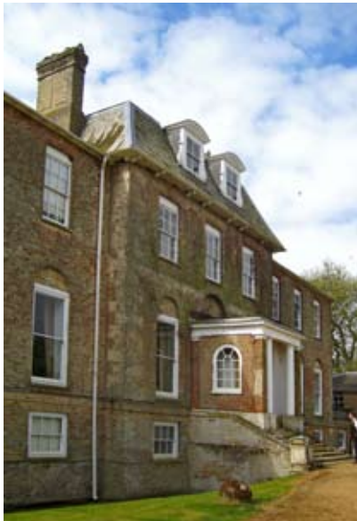
Above: Ryston Hall 1789 Entrance Front (publishers I & J Taylor, NWHCM: fineart\ tc15166.jpg)
