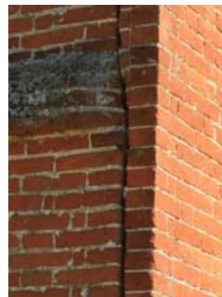
Westfield Farm showing the brick skin to a timber-framed building.
