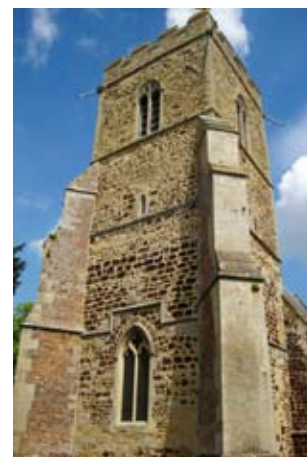
Holy Trinity, Stow Bardolph, clearly shows the use of different building materials.
