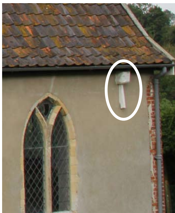
Above left: St Mary Magdalene, Withersdale, Suffolk Above right: interior showing reused tie beam with notches. Below: the anchor ties at either end of the tie beam (circled).
