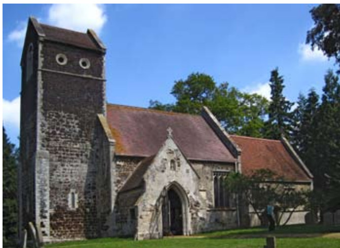
St Michael's Church, Ryston: lower part of the tower is medieval but the upper carstone is Victorian.
