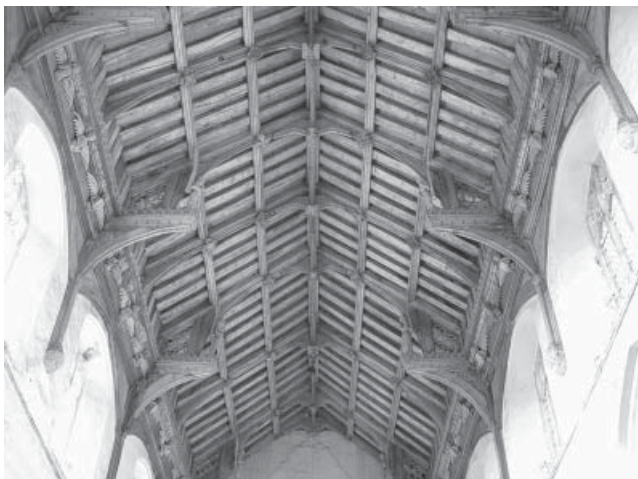
St Agnes, Cawston: hammerbeam roof.
