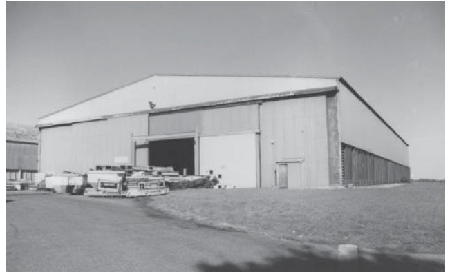
Photo 2: The ubiquitous type T2 ('Transportable') aircraft hangar. Over 900 were produced during the Second World War, and large numbers survive at airfields both operational and derelict. This one fares well in industrial use at North Creake, near Fakenham.
