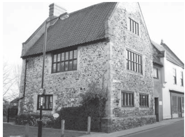
Stone House, Loddon. A late sixteenth century building using an array of building material with, most intriguingly, a generous show of freestone particularly on the quoins and around the windows.
