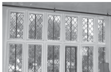
“Wide transomed windows of six to twelve lights were especially popular in the Elizabethan period and into the seventeenth century.” 5
