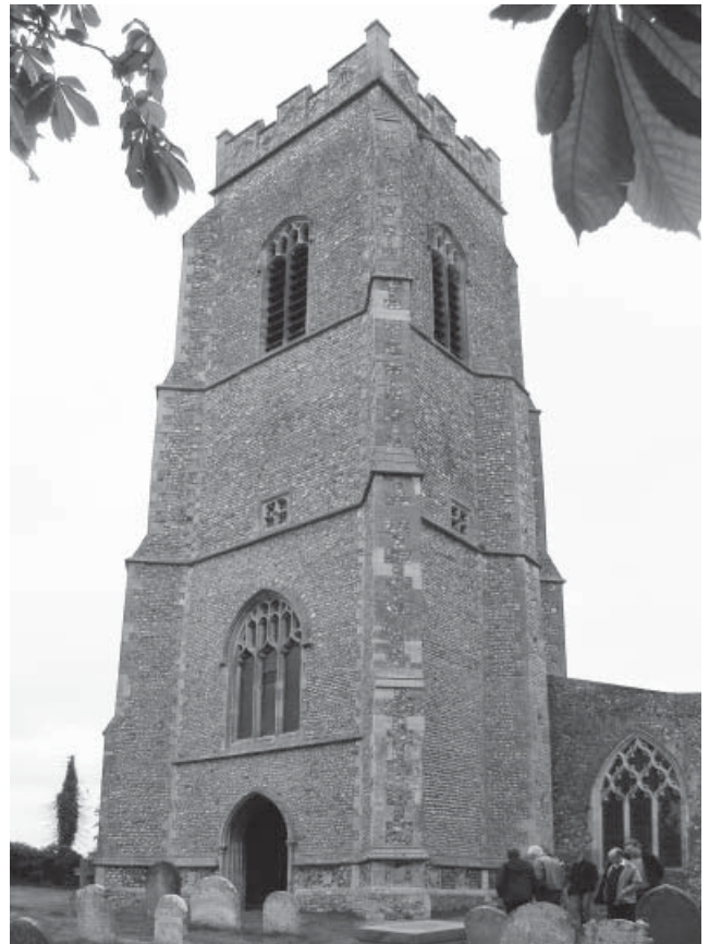
St Mary, Erpingham: a flint built tower.
