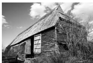
South west aspect of barn.
