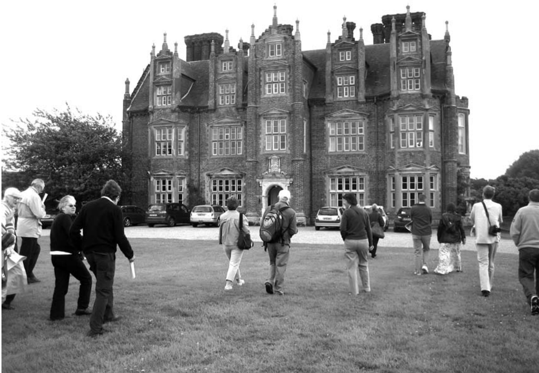
NHBG preparing to invade Barningham Hall approaching by the west facade. The early seventeenth century house has unusual double dormers. The oriel window protruding from the south face was an introduction by the Reptons in the early nineteenth century.
