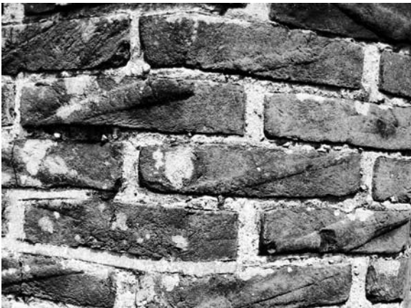
Diagonal skintling marks, mark of pre-mass production, on the brick polygonal angle porch buttresses.
