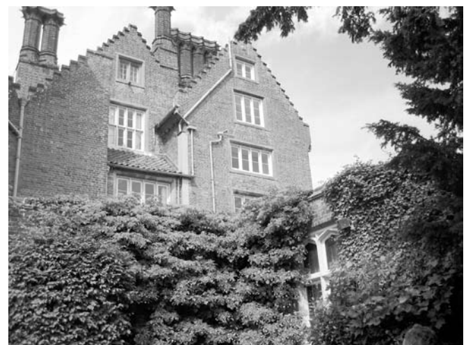
East facade with crowstep gables. Repton's kitchen is behind the greenery and the gun room to the right.
