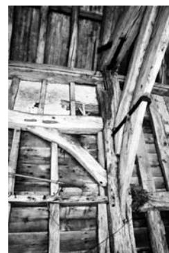
South east lintel
