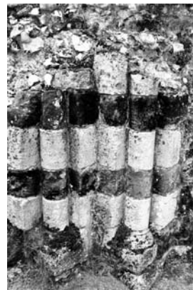
Priory church aisle piers used variegated materials for decoration, possibly with a Persian influence. (Photo: Rosemary Forrest)
