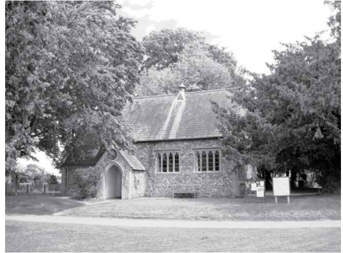
The attractive early nineteenth century church school at Welborne, now used as a community Hall.
