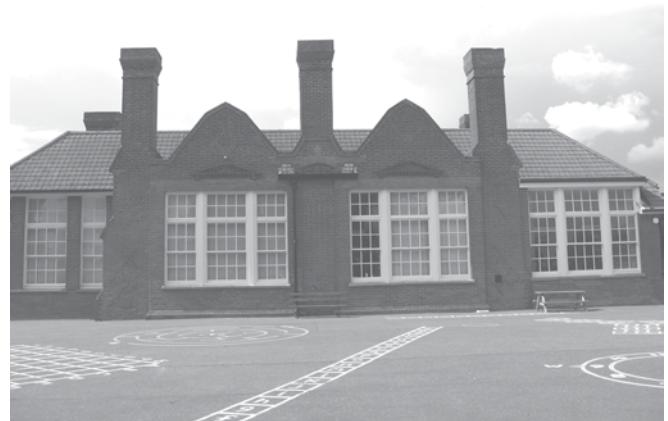
An unusual example of a new school built during the First World war at Swanton Morley demonstrating the value placed on light and fresh air as part of the educational philosophy of the time.
