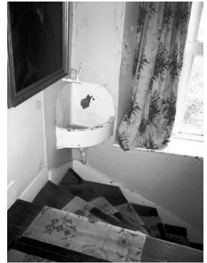
Early winder staircase with later wash basin.
