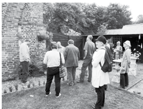
Inspection of a wall at Tydd St Giles
