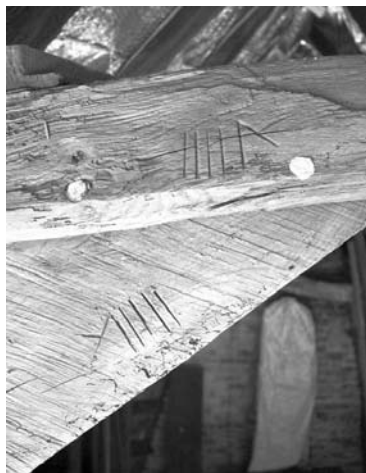
Chiselled marks on roof timbers.
