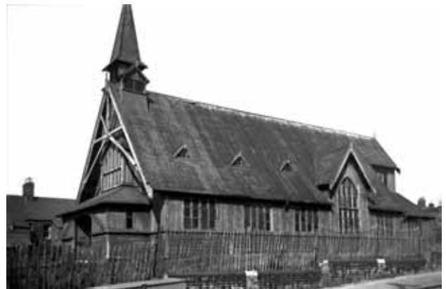
St Paul's, Magdalene Road prior to demolition in 1956. Photo from the George Plunkett collection by kind permission
