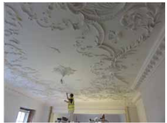
A new ceiling at Kilbooy, Ireland in 2010 1 Drawing 2 Casting 3 Installation
