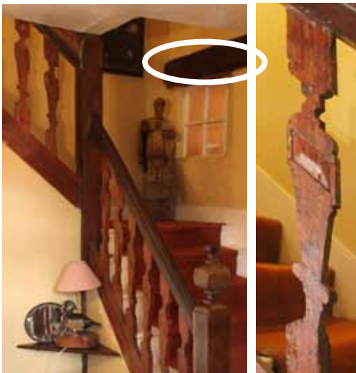
below right: baluster close-up
