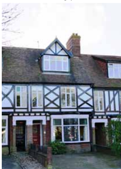
above: Concrete lintels and elaborate woodwork in Ceci Road - 1905
