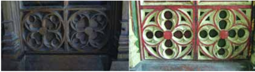
above: Figure 5. Dado base tracery from Barton Turf and Westwick rood screens.
