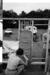
Timber frame showing the square panels used commonly in UK on the left. The thinner panels used in East Anglia on the right. Applying render to wattle and daub panel; clay pargetting attempts, after final render Richard Hyde admiring wattle and daub panel. NB only vertical wattle used, tied to horizontal ledges—East Anglian method
