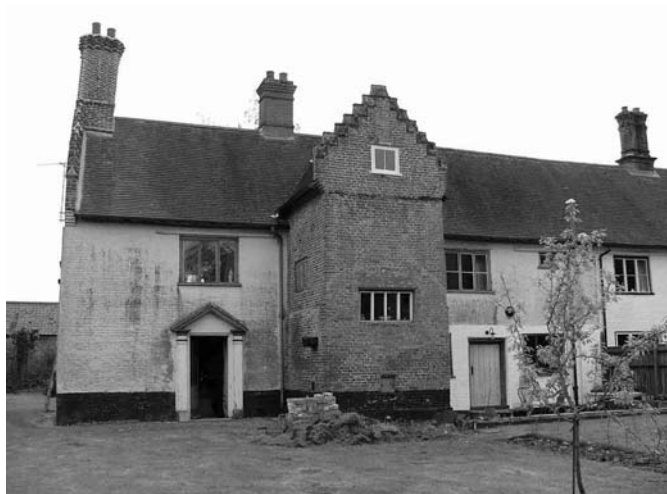
Ketteringham Hall Farm House Stair tower. Photo: Robert Limmer)
