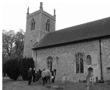
Norman masonry and blocked windows. (photo: Karen Mackie)
