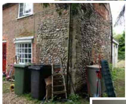
The western wrap-round gable with the reused stone from the Castle below: the truncated principal-rafter roof (photos: Michael Brown)
