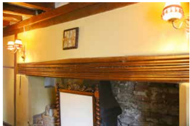
the moulded bressumer or mantle beam of the parlour fireplace
