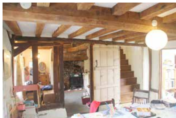
Looking west in the hall at the steep stairs and into the service-room extension
