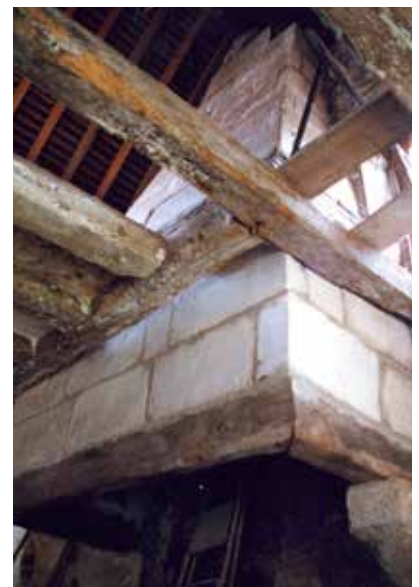
below: the completed chimney with the prominent new corbel
