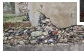
left: Two pieces of reused freestone in the walls, including a section of window mullion
