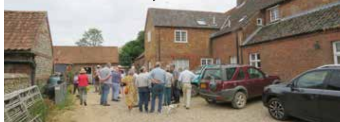
The rear of Burwood Hall Farm - a model farm of 1793 replacing the medieval Burghwood Manor; built inside the castle bailey.
