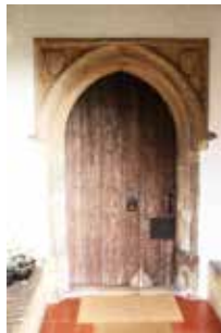
The 15th C doorway with decorated spandrels and an original plank and muntin door
