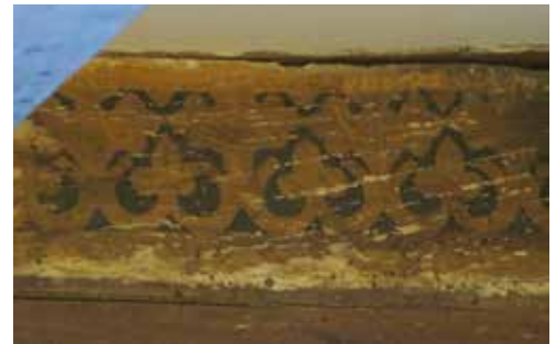
part of the decorative paint scheme on the parlour principal joist that must have been above the later ceiling (since removed) and therefore escaped being varnished over
