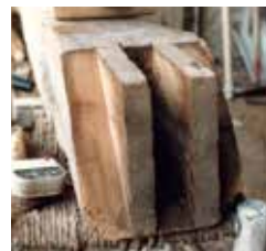
the new tenoned mitre
