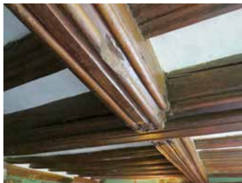
the moulded principal and common joists of the inserted hall ceiling
