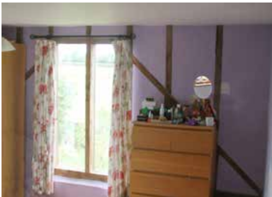
The thin, nineteenth-century, primary bracing
