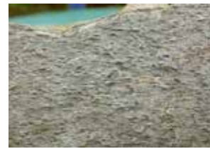
Sample 1 Schistose slate from the north face of the nave roof
