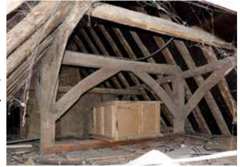
above) Queen Post roof - before c1550, a few until 1650. Used above open halls, but also in roofs above ceilings
