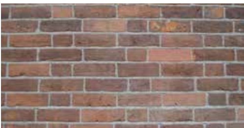
Flemish Garden Wall Bond - 3 stretchers, 1 header, 3 stretchers...
