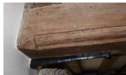
Sunk-quadrant chamfer with stepped run-out
