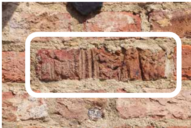
Probably the bottom row of the drying pile with impressions of straw
