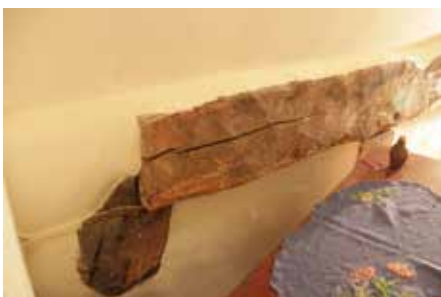
The scalloped effect of side-axe-prepared timber.
