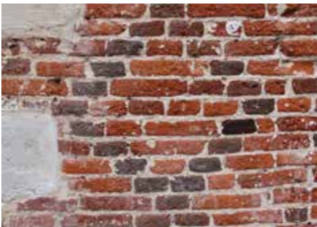
Decorative use of burnt bricks which were over-fired when bricks were often made in glorified bonfires rather than controlled kilns.
