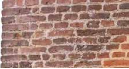
What shall we use next bond. The top two courses are not bonded at all
