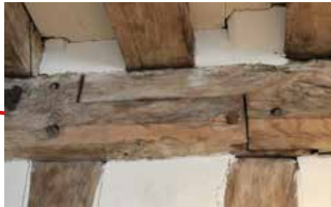
Short halving, longer bridle and 2 pegs (right) 1500-1600
