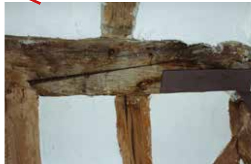
Splayed and under-squinted scarf . Up to 1600, little used after 1500
