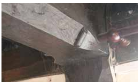
Run-out stop with bar
