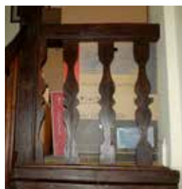
17/18C "Splat" balluster - many shapes, but just two dimensional
