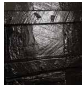
The angled saw marks of trestle-sawing, with a rarely-seen snap mark where the cuts met in the centre.
