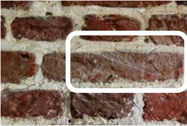
Bricks stacked in diagonal piles to dry, resulting in angled sagging between the bricks below
