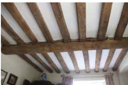
Laid flat, closely, C1500, -Litcham
