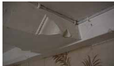
stepped runout with nick
