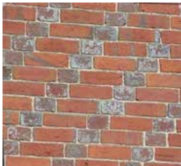
Still alternating headers and stretchers in each row, but the headers are placed above and below each other.
