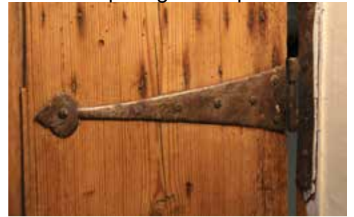
strap hinge on a plate
