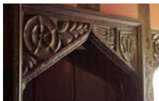
Spandrelled doorway into the service chamber, Yew Tree Farm, Fornsett (often just plain)
