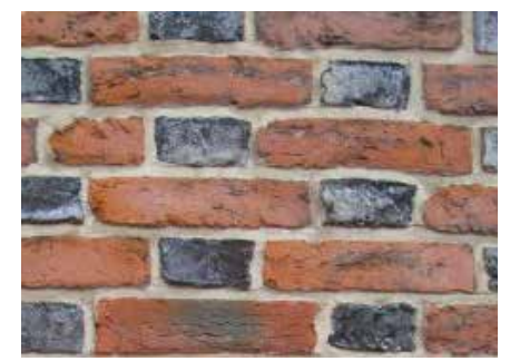
Decorative use of burnt bricks which were over-fired when bricks were often made in glorified bonfires rather than controlled kilns.
