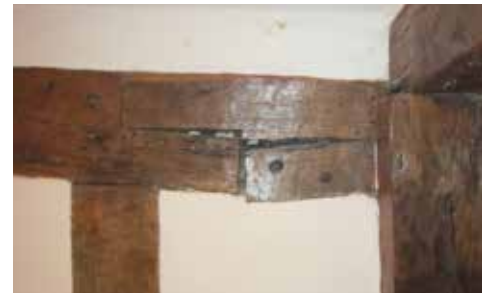
Splayed and under-squinted scarf . Up to 1600, little used after 1500
