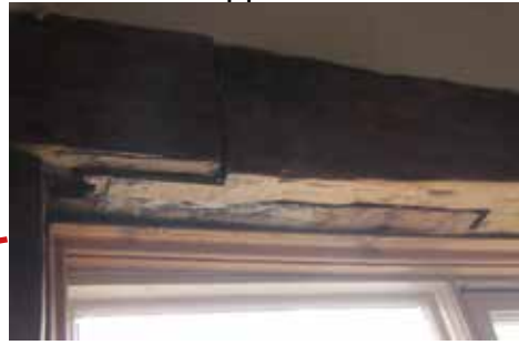
Face-halved scarf 1550 on
