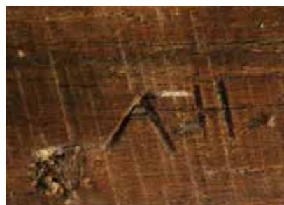
The almost vertical saw marks of pit sawing.
