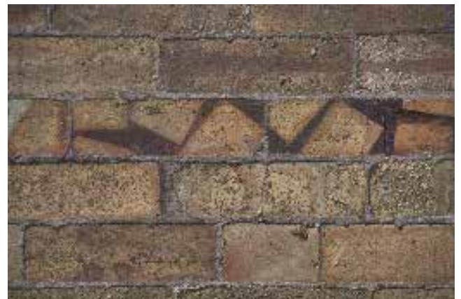
Even modern bricks overcook sometimes, leaving images of the bricks stacked above or below them in the kiln
