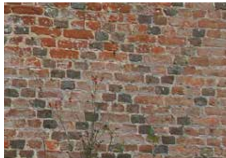
Decorative use of burnt bricks which were over-fired when bricks were often made in glorified bonfires rather than controlled kilns.
